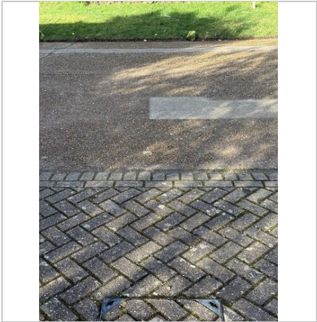
Main manhole opposite camera head 02 Mar 2026 09:55
