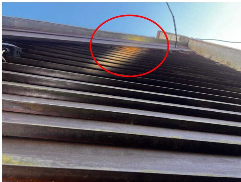
Figure 3. Gaps between the wooden cladding
