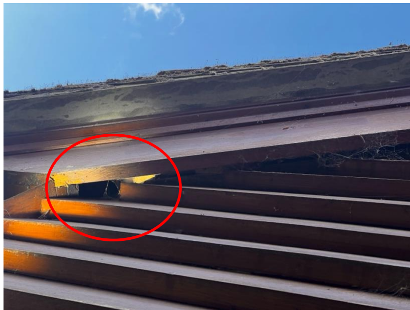
Figure 5. Ingress points noted on southern elevation
