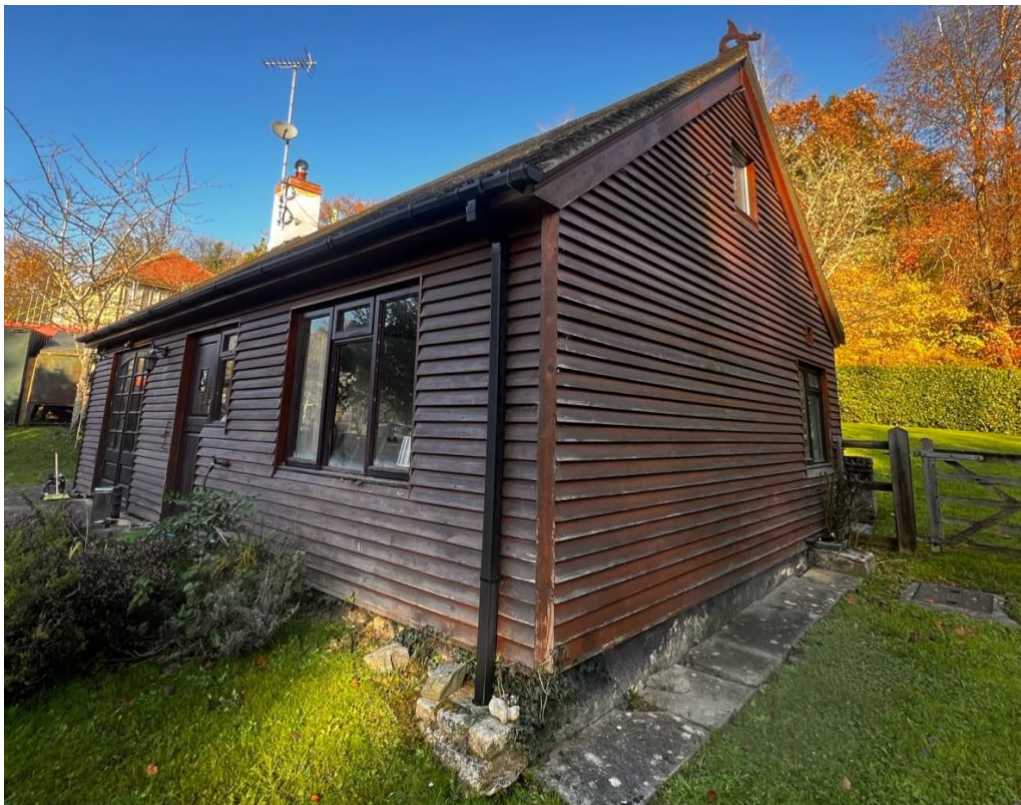
Figure 2. Wooden cladding on all elevations
