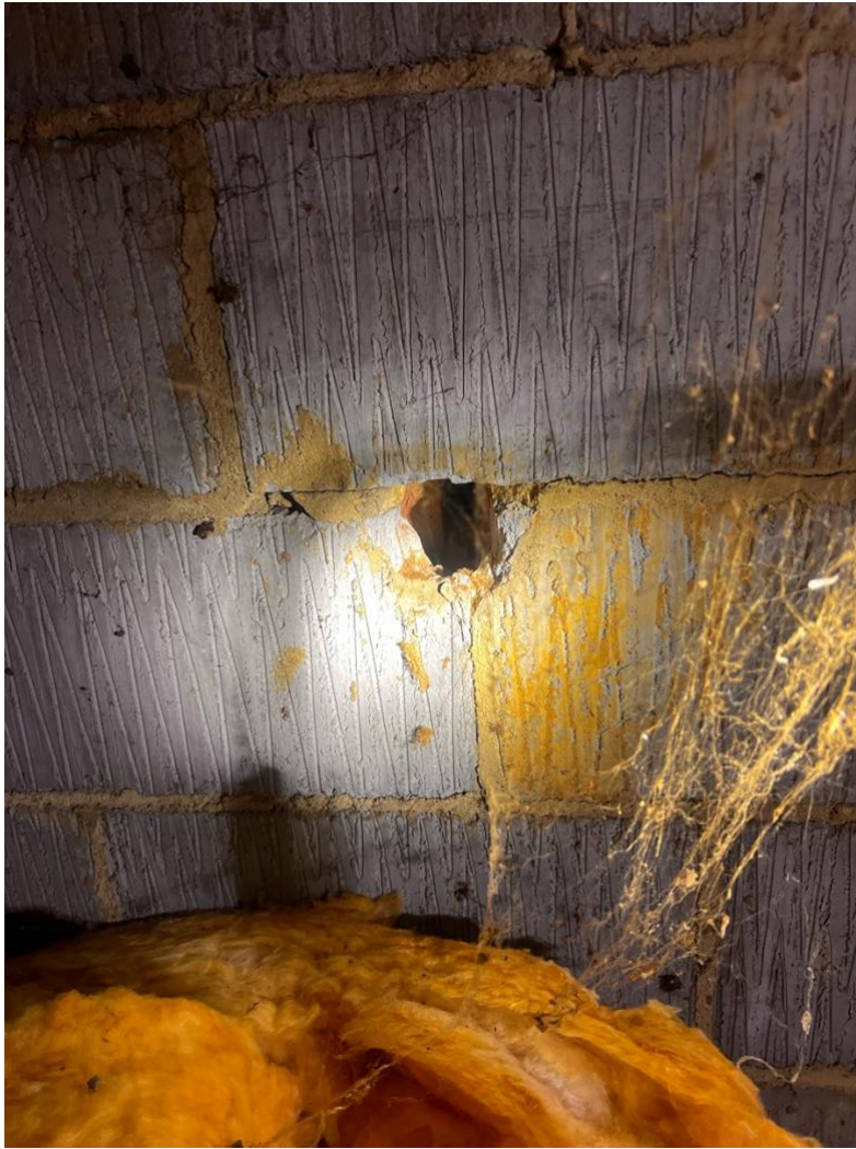
Figure 9. Ingress point noted (eastern gable end)
