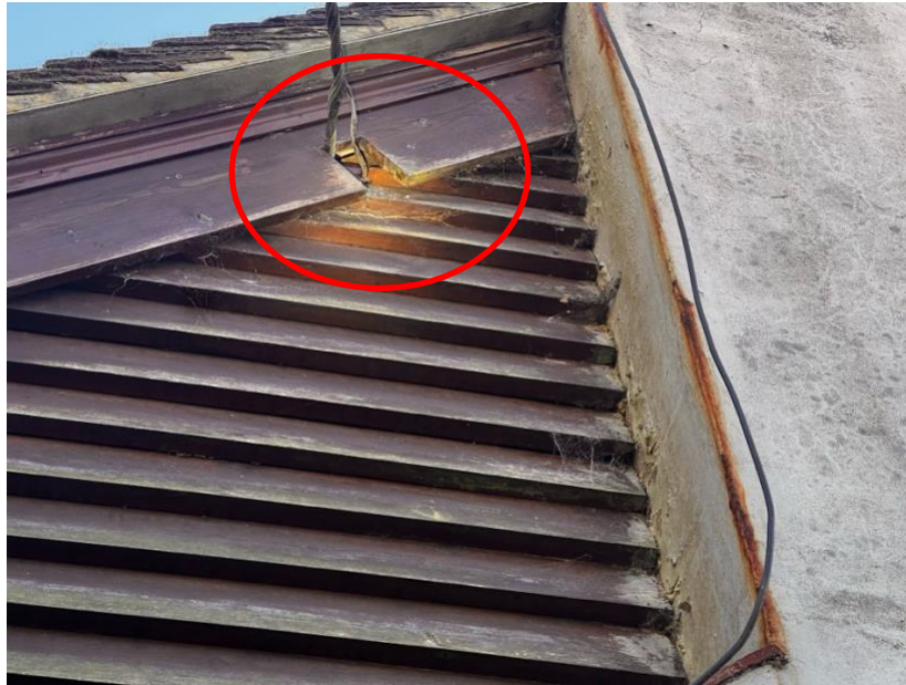
Figure 4. Gap within the wooden cladding
