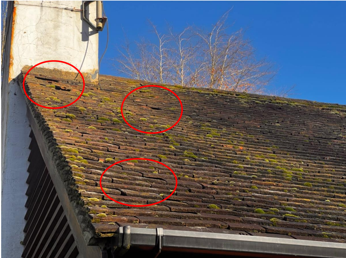
Figure 6. Gaps between concrete tiles (southern elevation)
