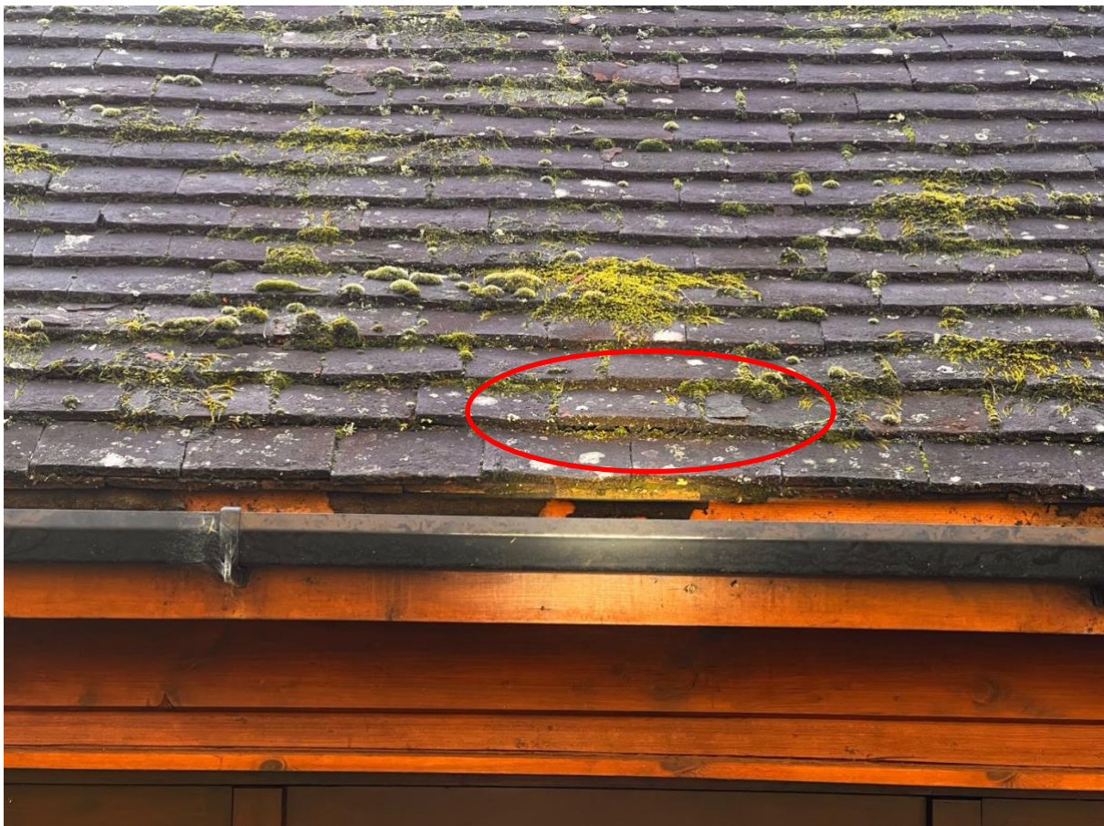
Figure 7. Gap between the roof tiles (northern elevation)
