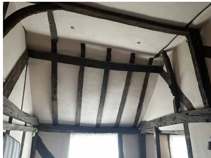
First Floor - historic timber frame roof
