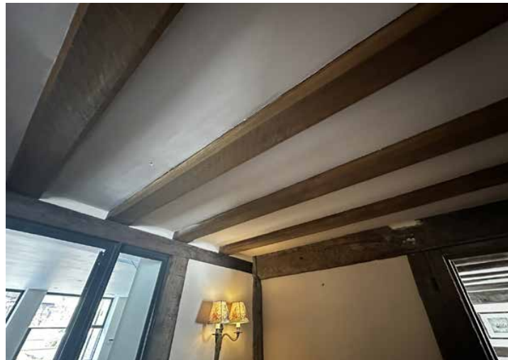
Ground Floor - new timber framing on the Ground Floor ceiling (infilled void above removed staircase)
