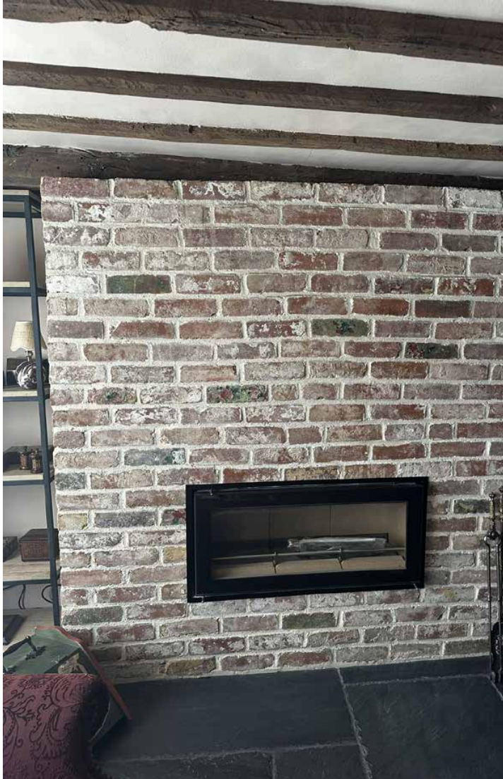
Ground Floor - New fireplace in north-eastern living room with reclaimed bricks from collapsed bake house
