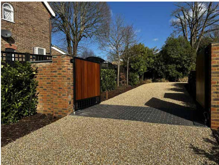
Gravel driveway and new gates
