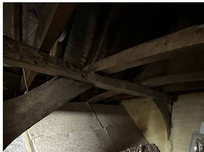
Attic - historic timber frame roof
