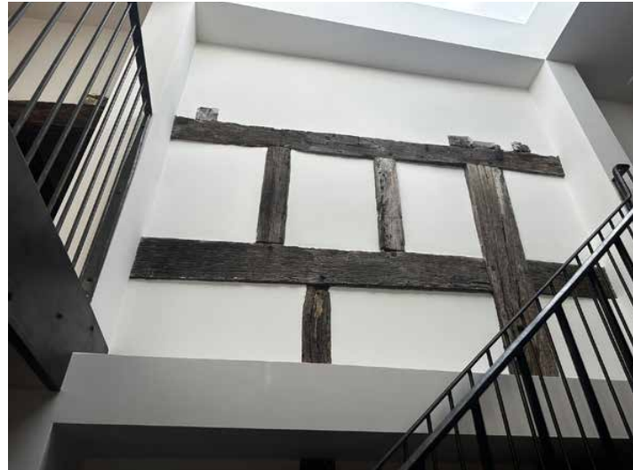
Historic timber frame wall in stairwell
