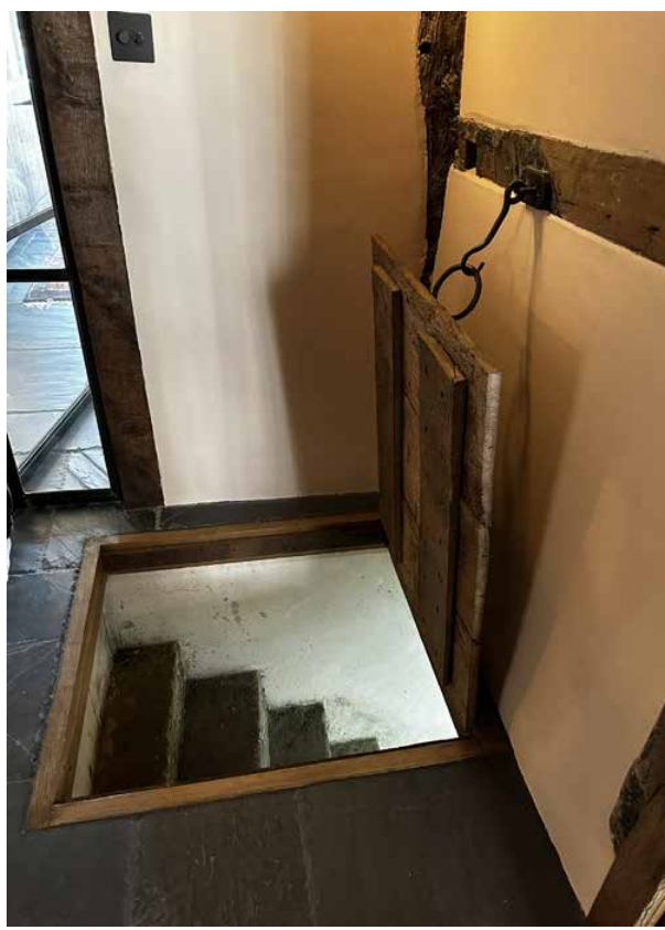
Ground Floor -access hatch to basement
