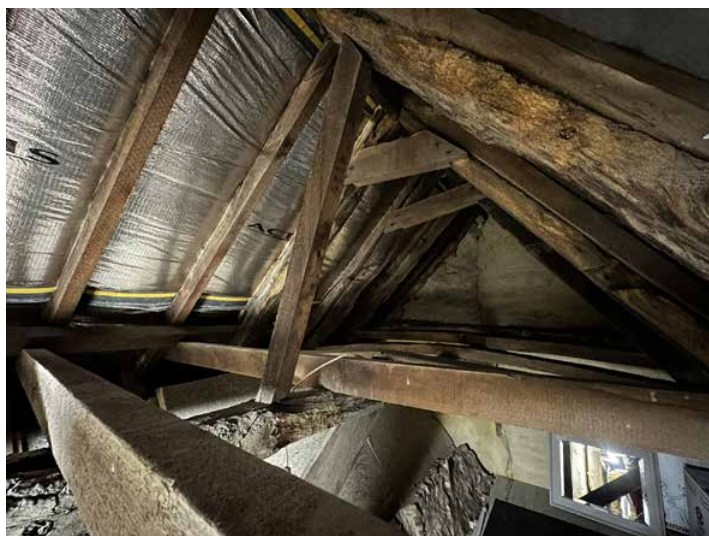
Attic - historic timber frame roof
