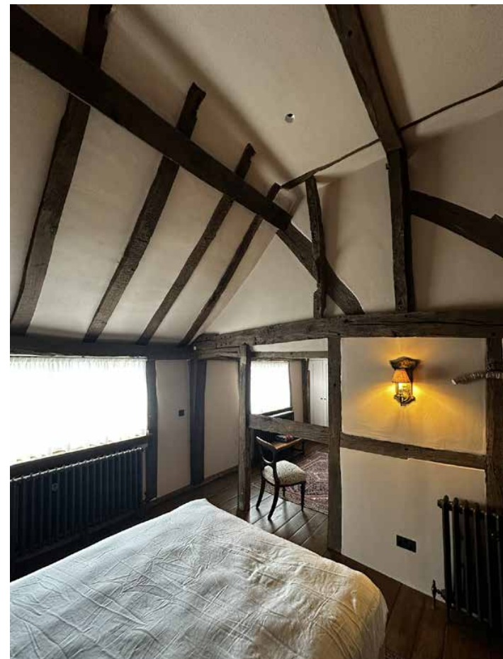
First Floor - historic timber frame roof
