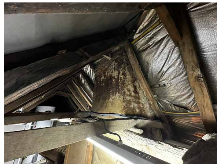
Attic - historic timber frame roof
