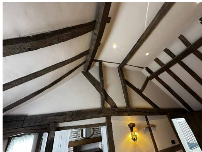
First Floor - historic timber frame roof
