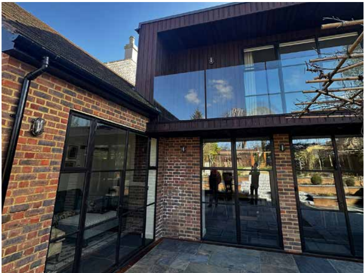
Rear elevation & re-constructed bake house
