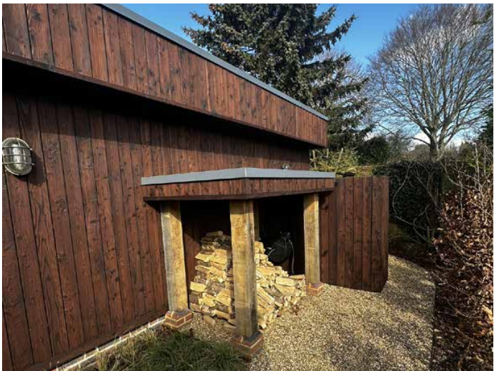
Covered loggery and irrigation tank enclosure adjacent to the garage
