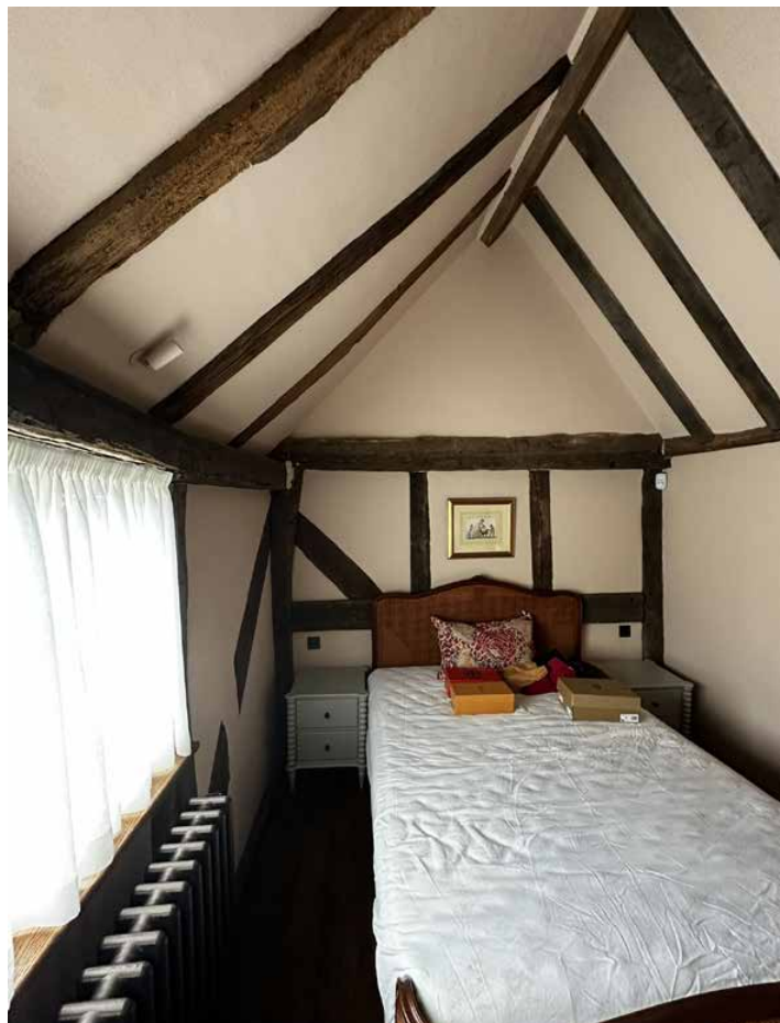
First Floor - historic timber frame roof
