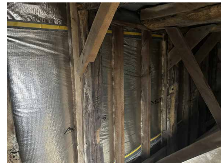
Attic - historic timber frame roof, new insulation
