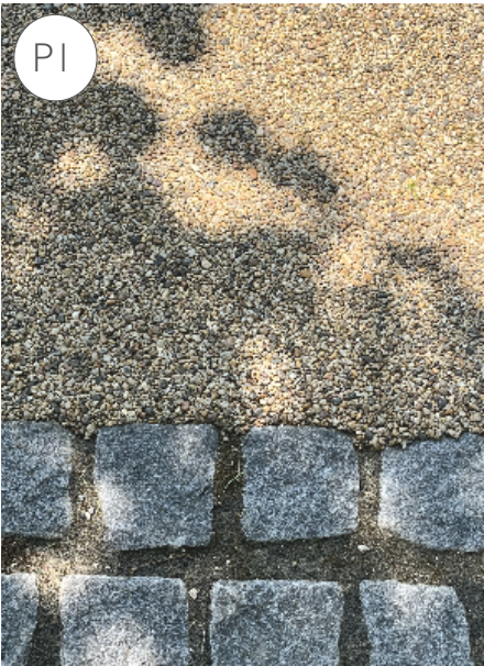
PERMEABLE RESIN / HOGGIN AND SETTS
