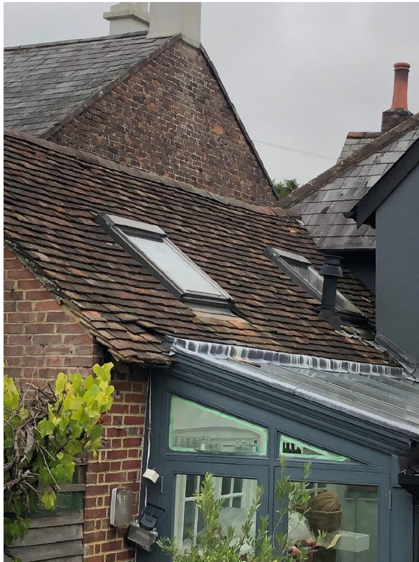
Figure 31: Bake House roof (south slope) as seen in 2022 with 2 no. modern Velux rooflights. Source: Gould Baxter Condition Report
