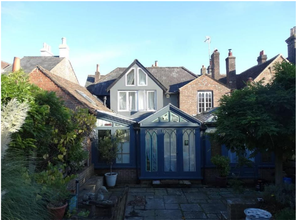
Figure 7: Marlow House, west elevation, prior to the commencement of the scheme as implemented
