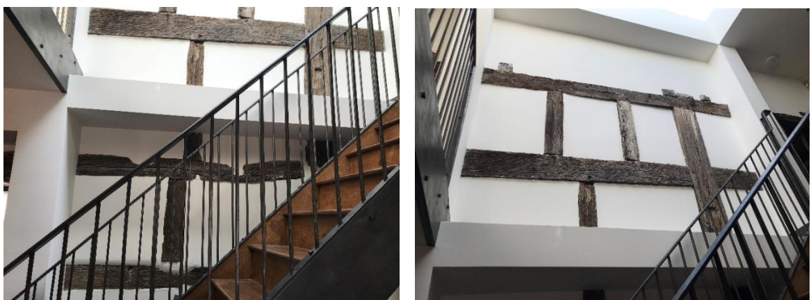
Figure 39: Box framing to west wall of the 15 th century house with internal windows infilled with wood wool panels and lime plaster.
