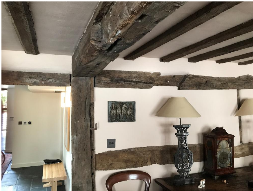
Figure 12: main E-W ceiling beam to the living room showing the location of an original partition and doorway adjacent to the northwest wall. The timber jamb post and stud partition is proposed to be reinstated.
