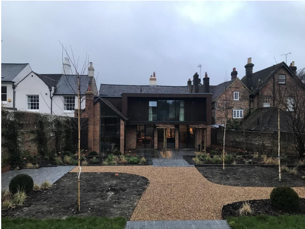
Figure 33: View of Marlow House from the rear garden (west). Note the prominence of the restored 15 th century roofscape compared to the prior situation shown at Figure 7.
