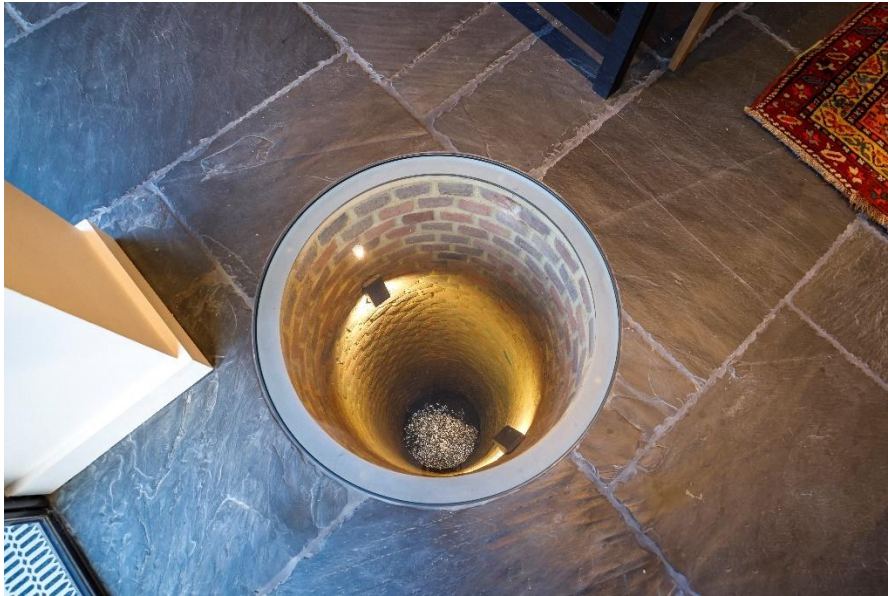
Figure 32: Rediscovered well shaft (re-lined in handmade brick) and groundwater storage chamber within the kitchen area. See DAS for images of well as revealed and during construction phase
