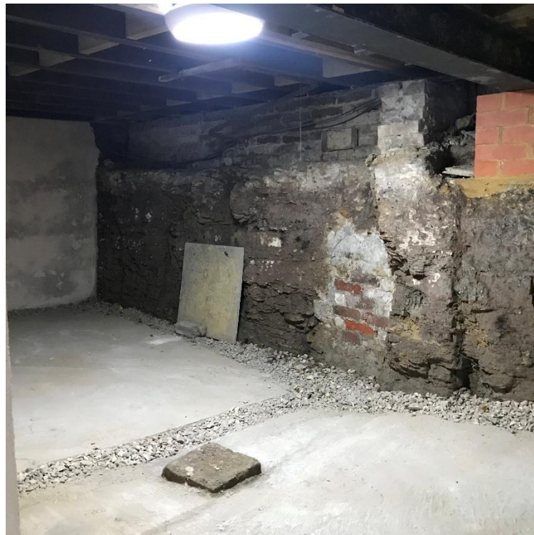
Figure 36: Renewed steel beam with new noggings and joists at basement level. The pre-existing concrete floor has been augmented by a French drain and brick walls coated with breathable hydraulic lime render to regulate the damp.
