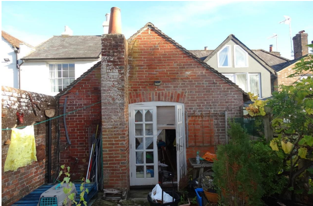
Figure 18: View of the former Bake House from the west prior to dismantling. Source: Desbruslais Chartered Surveyors Statement of Heritage Significance of 13 th October 2022
