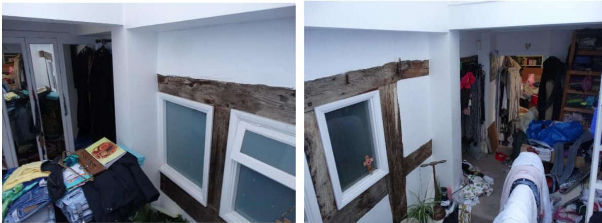
Figure 29: Box framing to rear (west) wall of the 15 th century house with internalised modern timber casement windows. Source: Desbruslais Chartered Surveyors Statement of Heritage Significance of 13th October 2022
