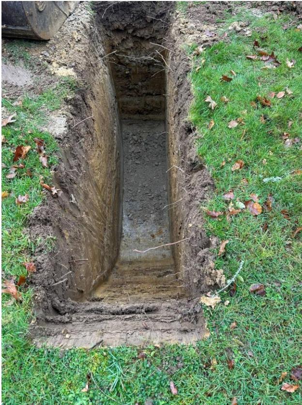
Figure 3.4 Slip Trench A
