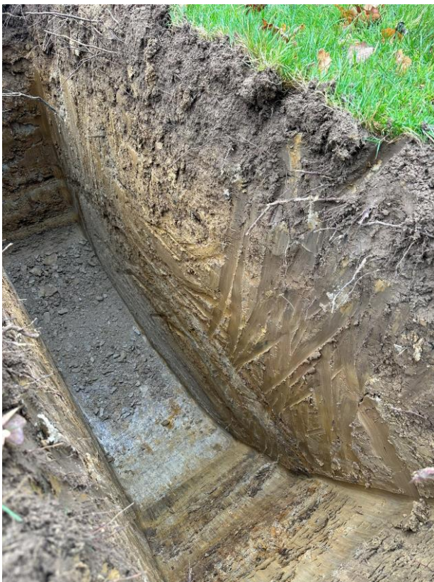
Figure 3.4 Slip Trench B
