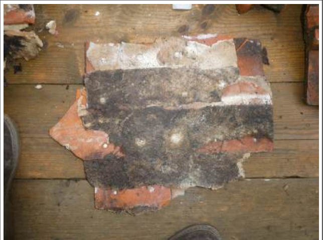
Roof View One (6)
