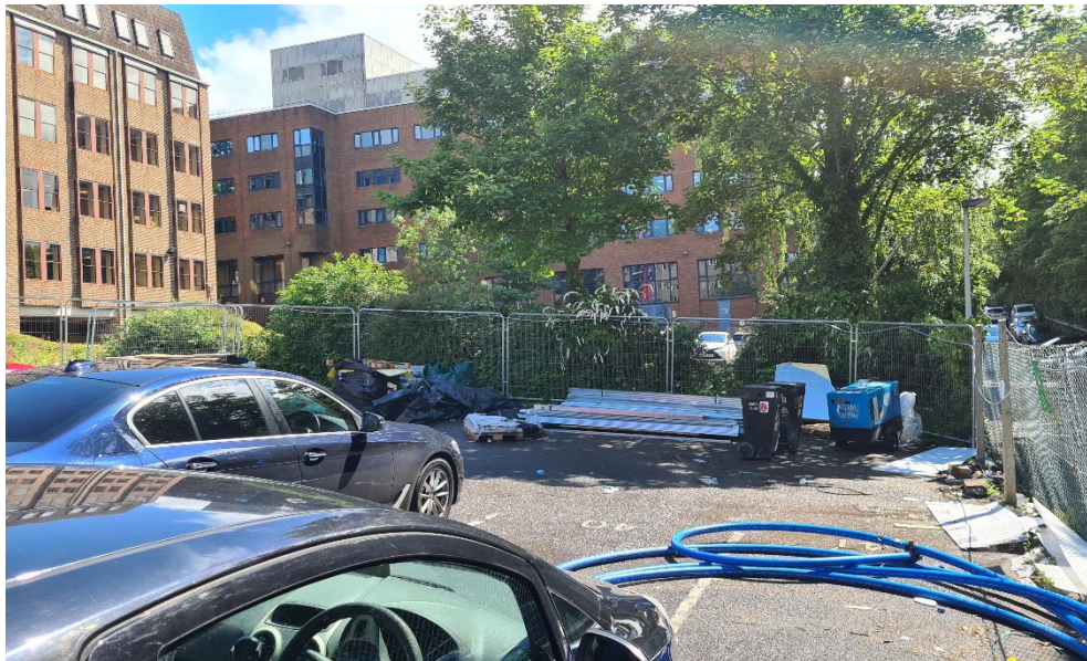
2. View of lower part of car park looking at the soakaway on the south west corner of the site (June 2022)
