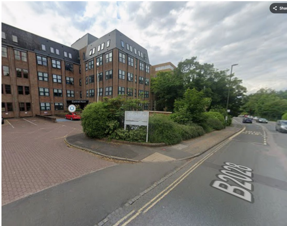
1. Front view of the site (Central House) – From Google maps (June 2024)
