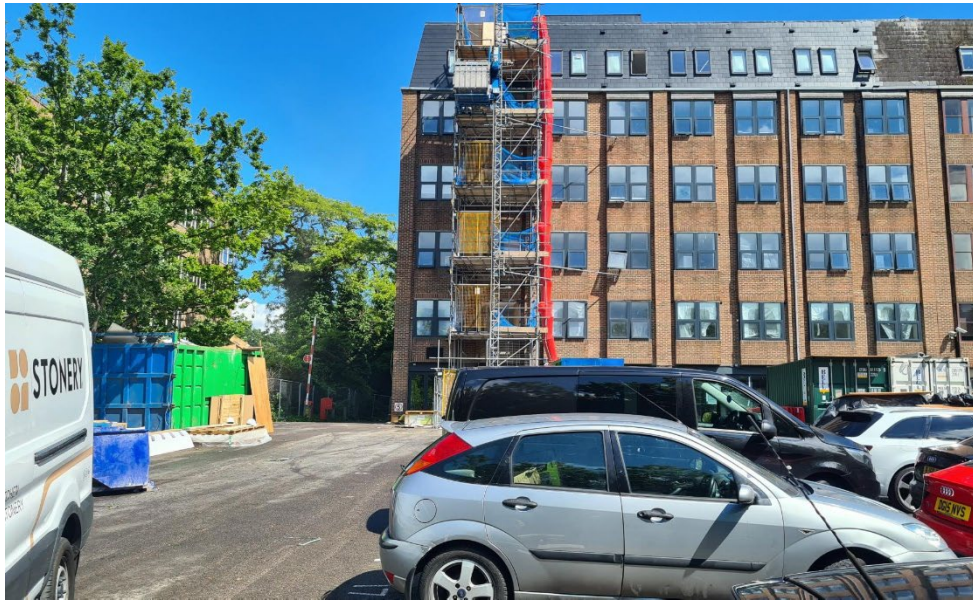
5. Looking east towards central house from the lowest part of the site (June 2022)
