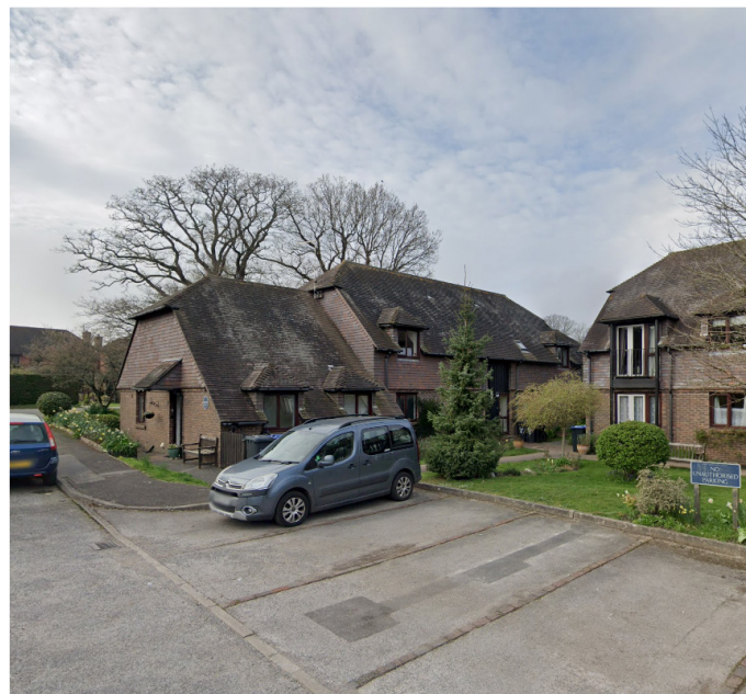
1 - 1 Paynesfield - Brickwork and Tile Hanging
