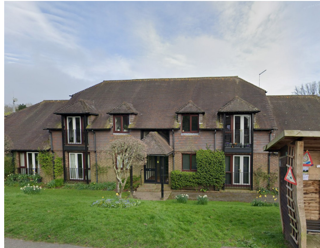
3 - 35 The Street Bolney - Dormer windows flush with external wall.
