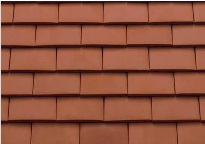
Roofing - Clay Tiles
