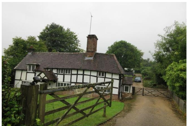
Figure 18: Yew Tree Cottage (Grade II).
