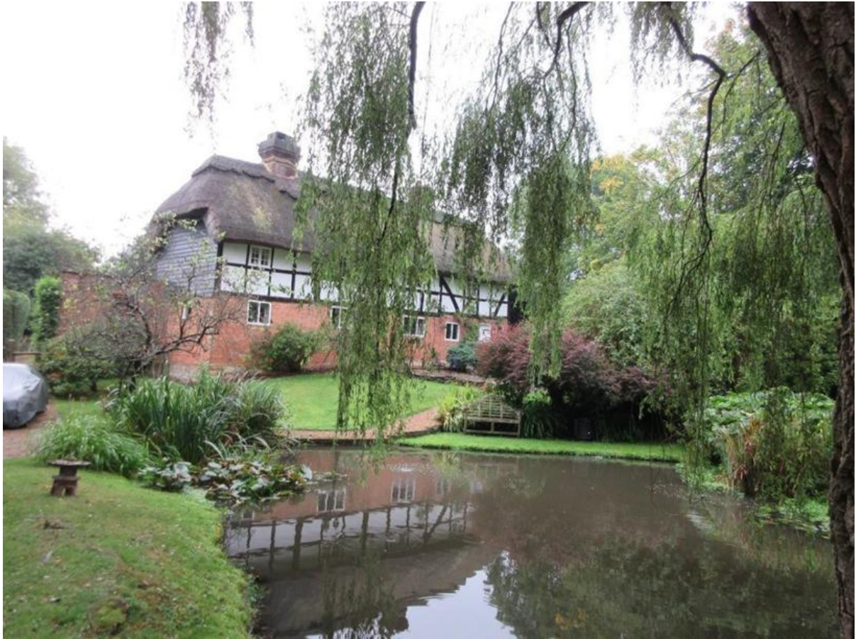
Figure 17: The Thatched House (Grade II).
