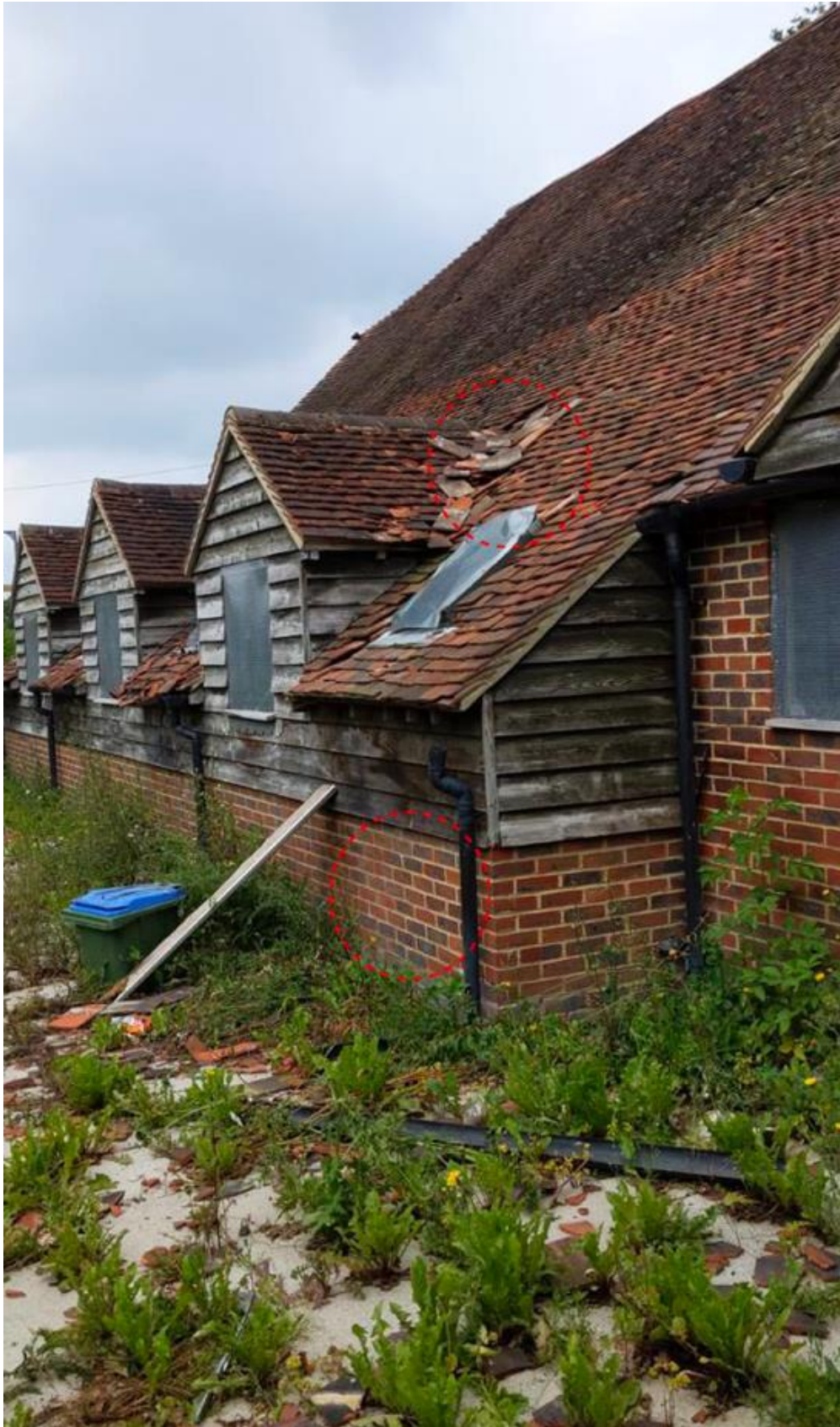
Southern elevation of Lowlands Farm Barn showing lean-to extension
