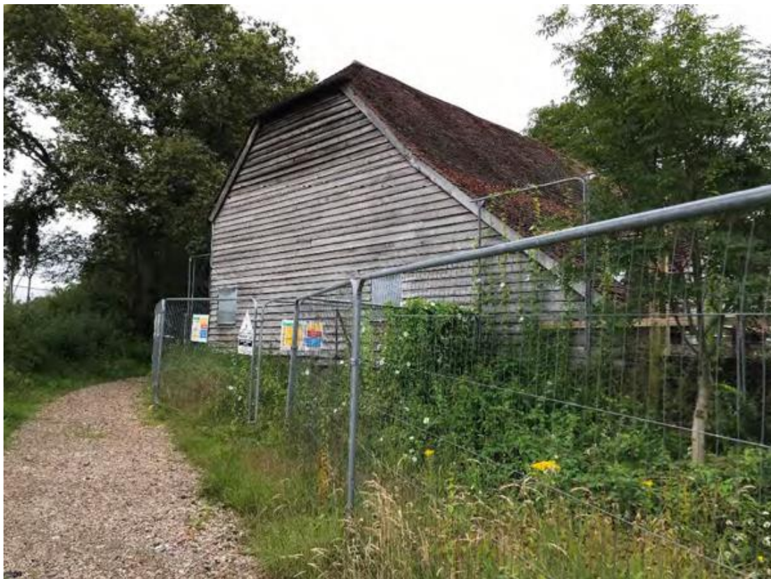
West elevation of Lowlands Farm Barn from Freeks Lane
