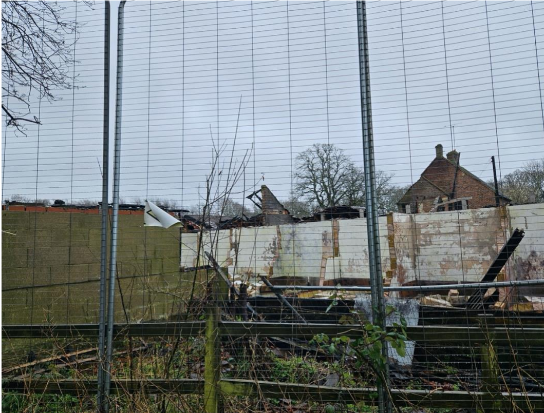
View of Lowlands Farm Barn looking south from Freeks Lane
