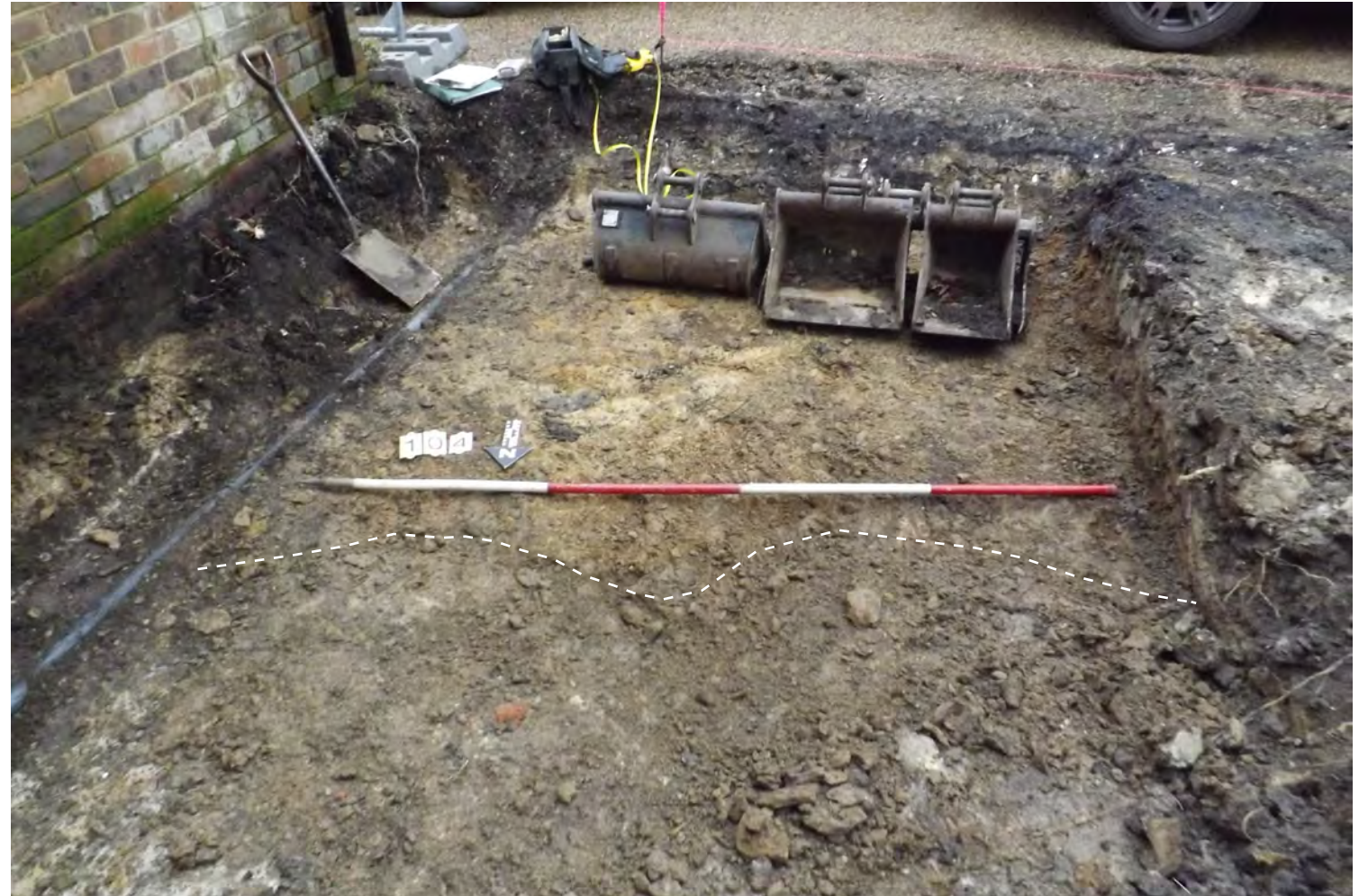
Southern edge of Cut 104 (highlighted in white), within southeast corner of excavation (machine buckets are resting upon the geological horizon)
