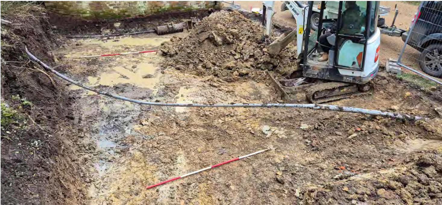
View to the southeast of site excavated down to formation level (spoil stored on previously monitored area)
