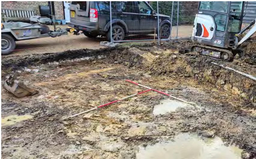
View to the southwest of site excavated down to formation level
