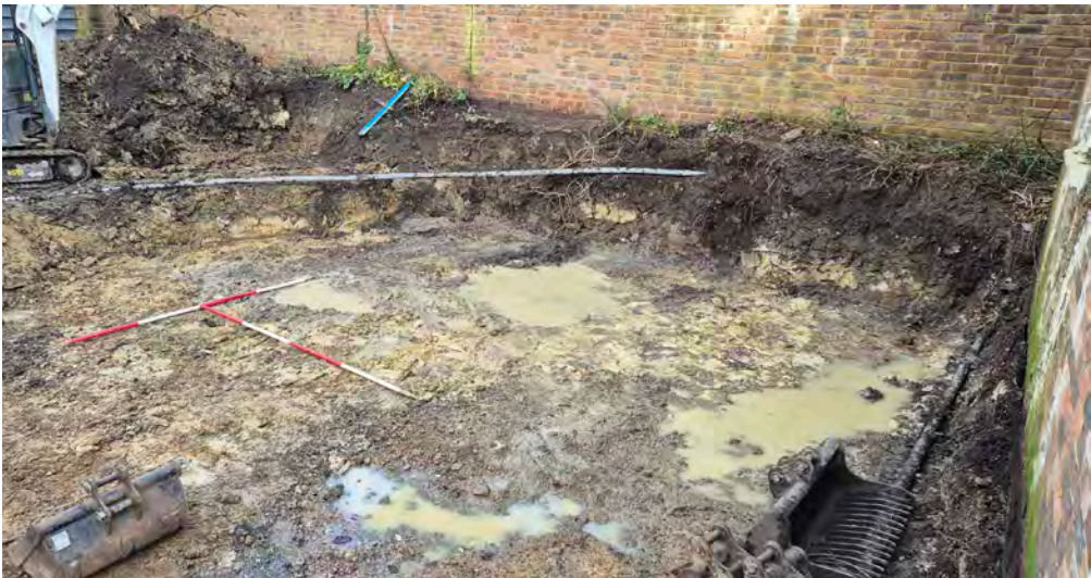
View to the northwest of site excavated down to formation level
