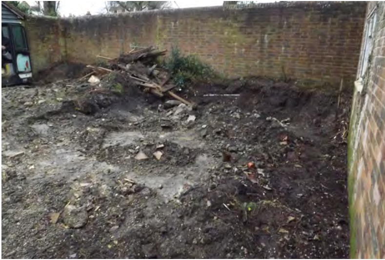
View to the northwest of site after initial clearance
