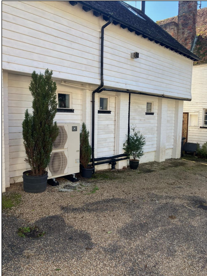
Figure 3 - View of ASHP installation
