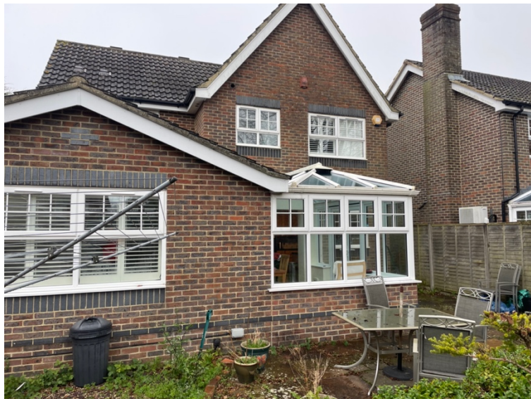
View looking north-east showing rear elevation
