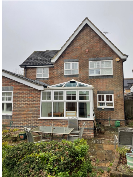
View looking north showing rear elevation
