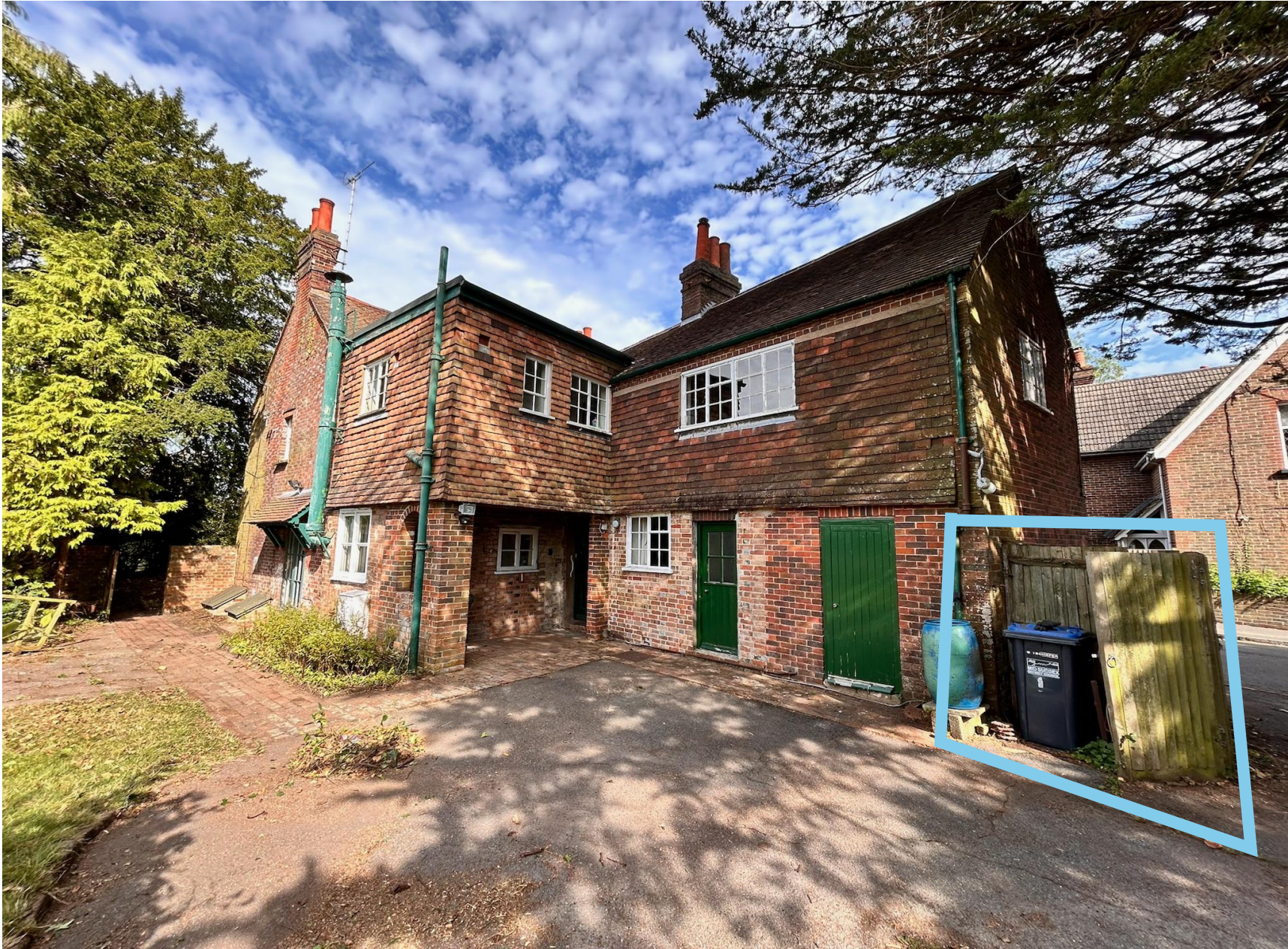
Picture taken by applicant on 24/08/2024 with existing 1800 mm closed-board fence and gate highlighted
