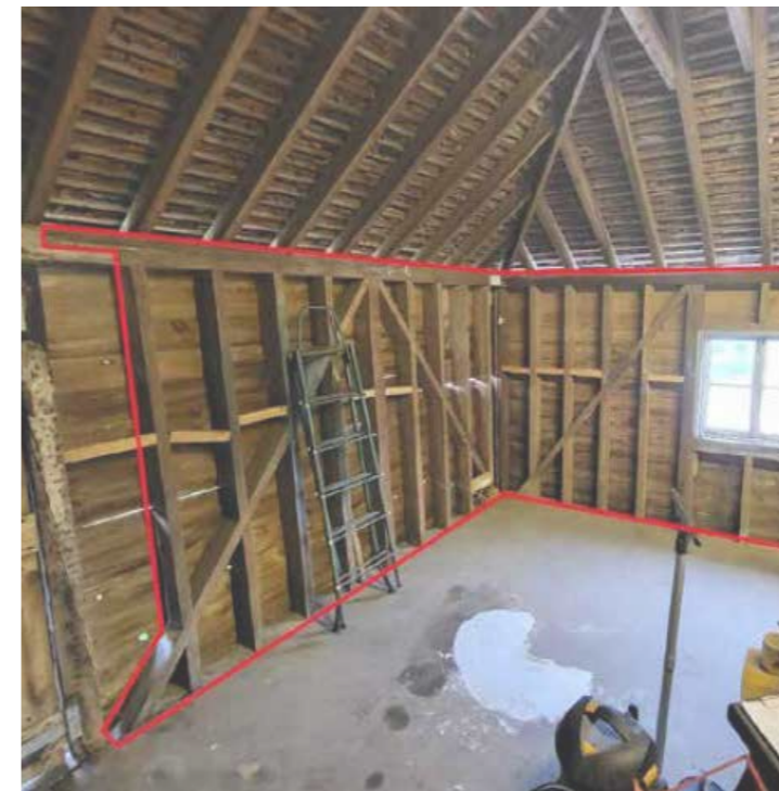
Internal photograph highlighting replacement timbers
