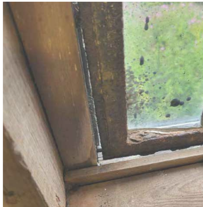
Internal photograph showing poorly fitted windows
