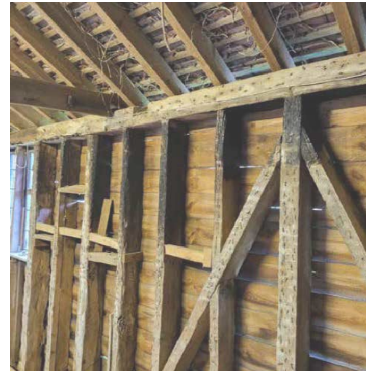
Internal photograph showing fire damage
