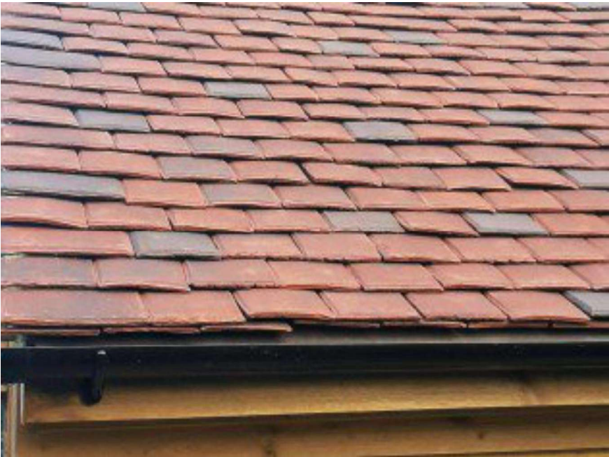
Tudor Restoration roof tiles
