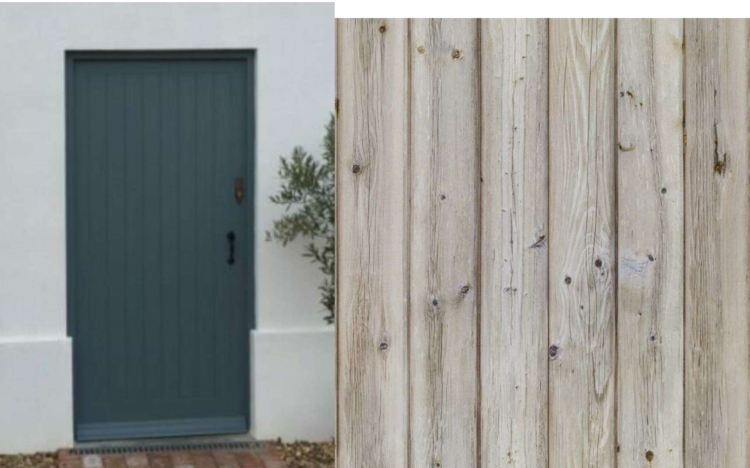
Painted timber framed doors and windows
