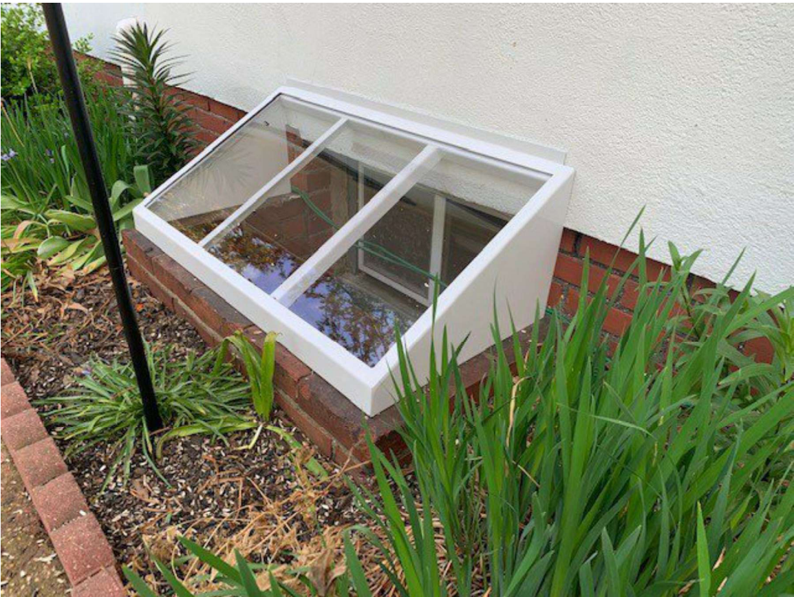
Well painted timber glazed cover
