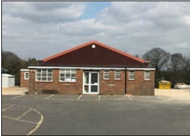
Photograph 2. The front (southern elevation) of the light industrial building to the south of Land North of Borers Arms Road.
