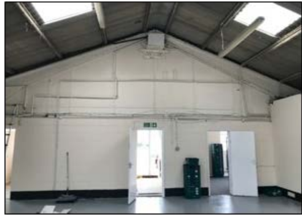
Photograph 3. An interior space of the light industrial building showing natural light and lack of enclosed loft space.
