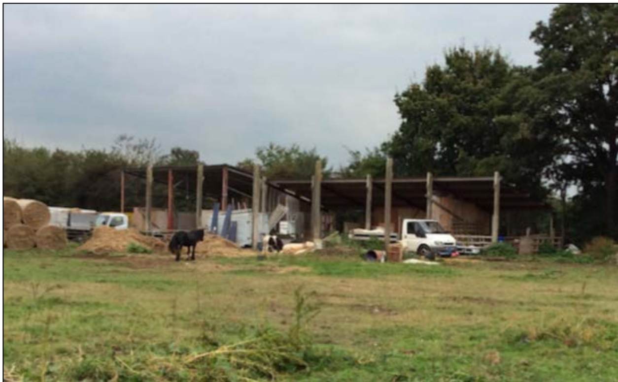
Photograph 1. A view of the agricultural building on Copthorne Bank.
