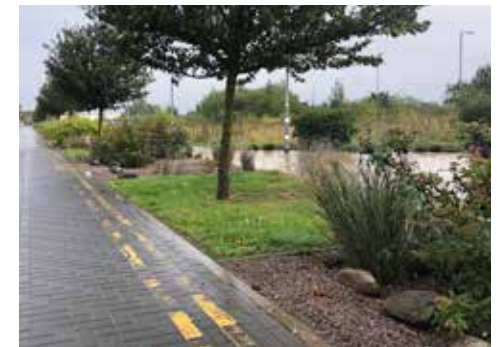
Wetland planting with crushed aggregate along roadside. (Cambridge North Station Source: James Dee / AECOM 2023)
