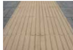
Corduroy Paving in buff
