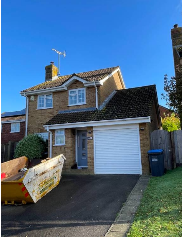
Photograph 1 – Taken from the road at the front of the property during the survey.
