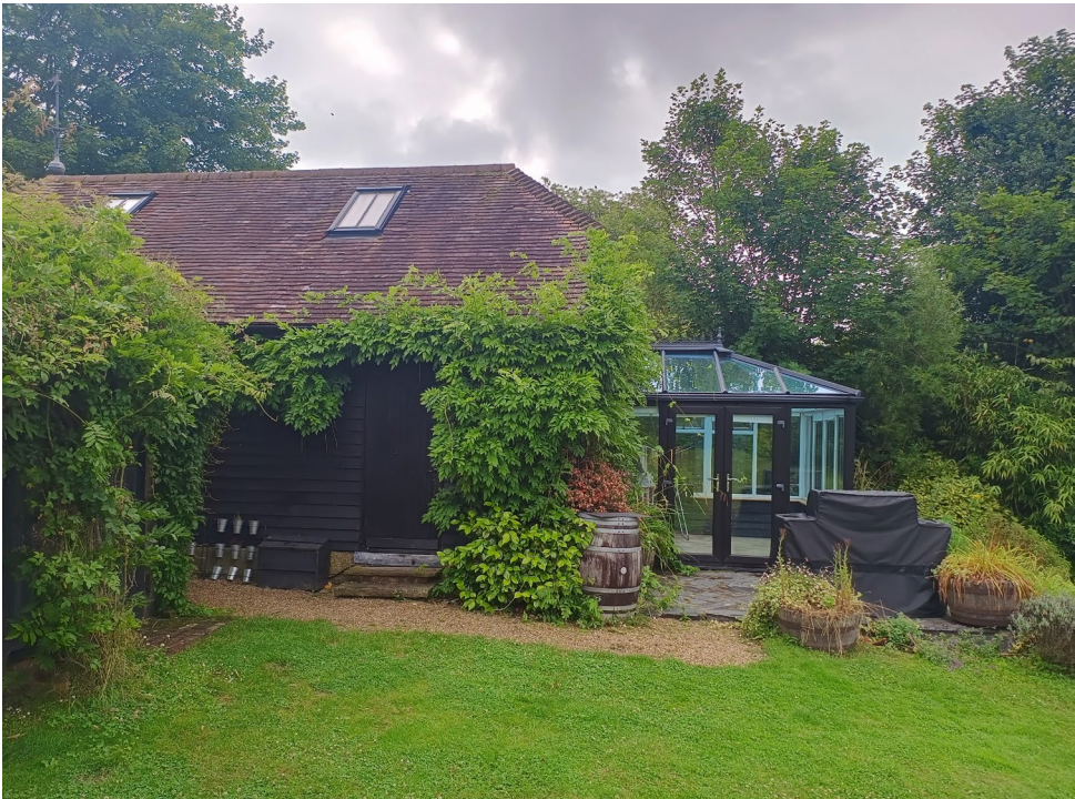
West Elevation of Garage
