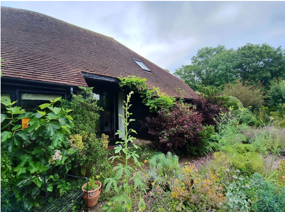
South Elevation of Main Barn
