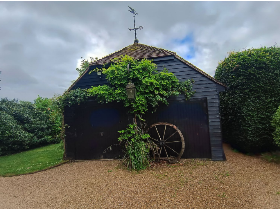
North Elevation of Garage
