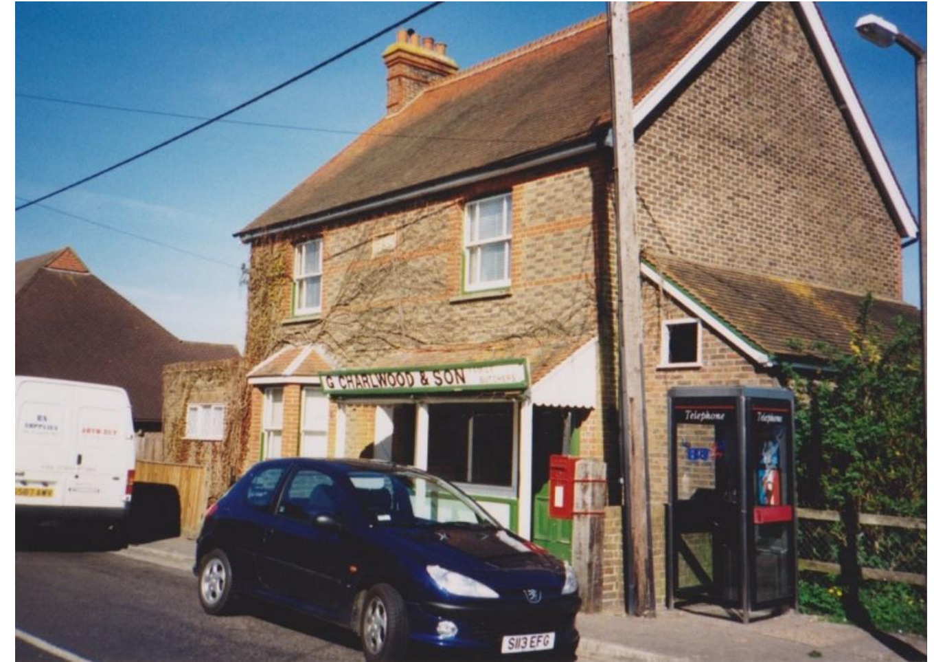
A view of G.Charlwood & Son shop front signage, viewed from the SE.
