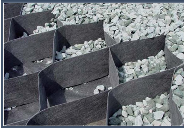
Figure 12 Examples of Cellweb filling with angular stone
