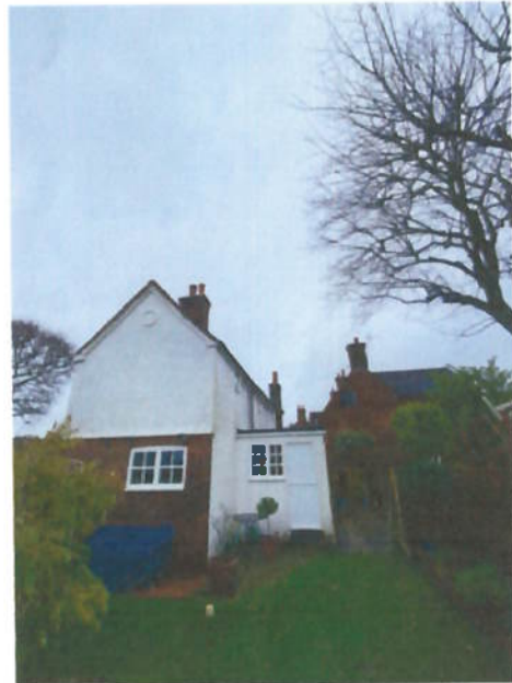
Image showing current crown clearance between T1 and the existing cottage.
