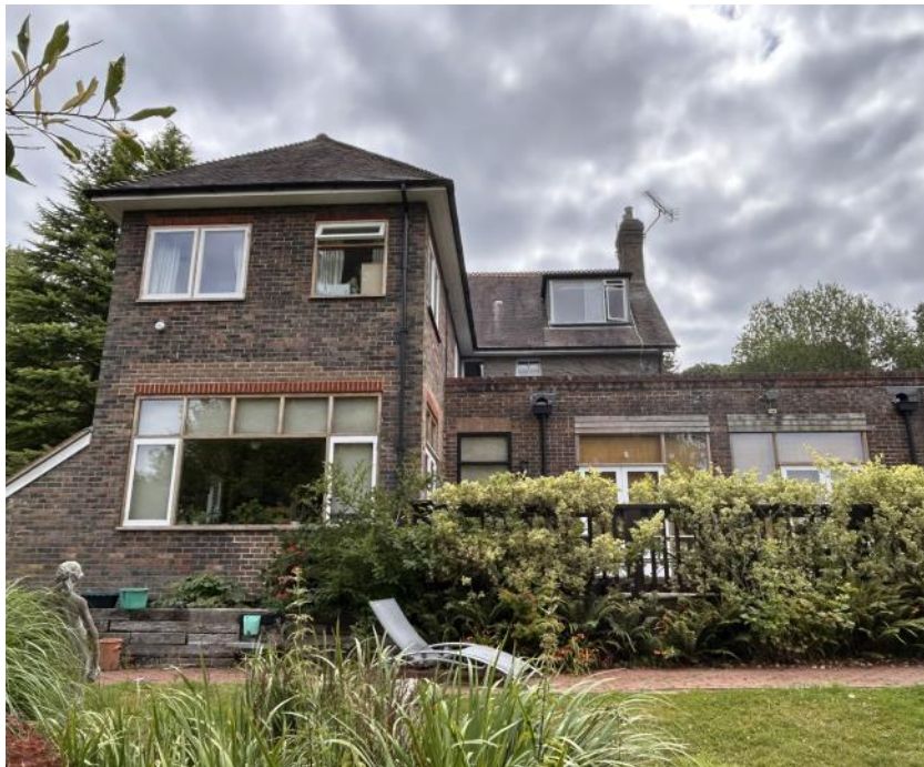
Rear of house from garden from the South West
