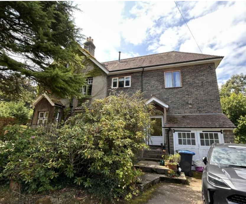
Driveway approach to Oak Lodge with side entrance to Kitchen.
