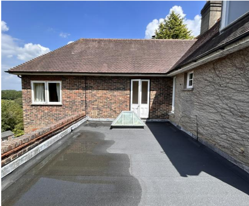
First floor flat roof
