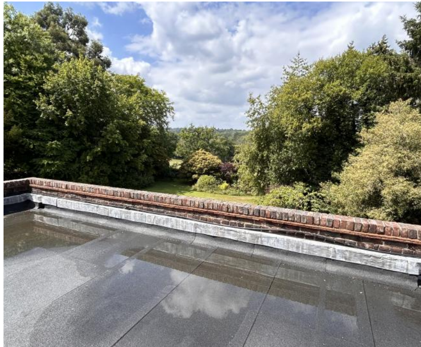
View to the South West from the first floor flat roof.
