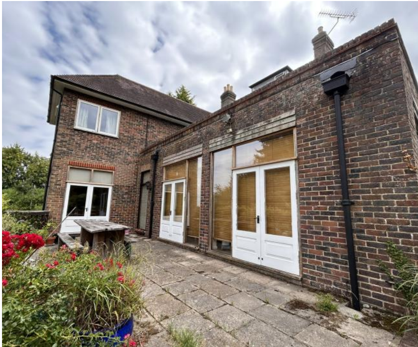
Rear of house at Ground Floor level.
