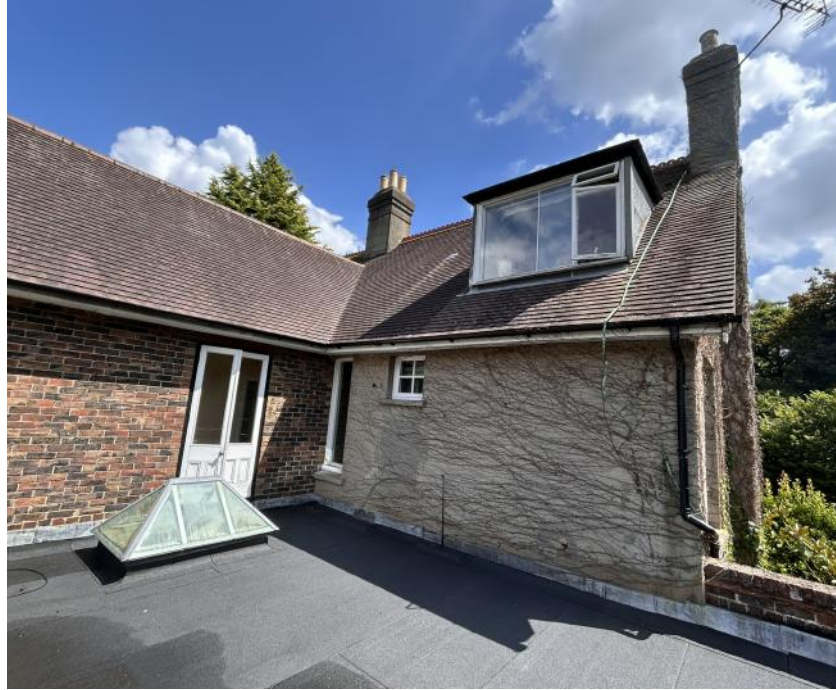
First floor flat roof with existing box dormer above
