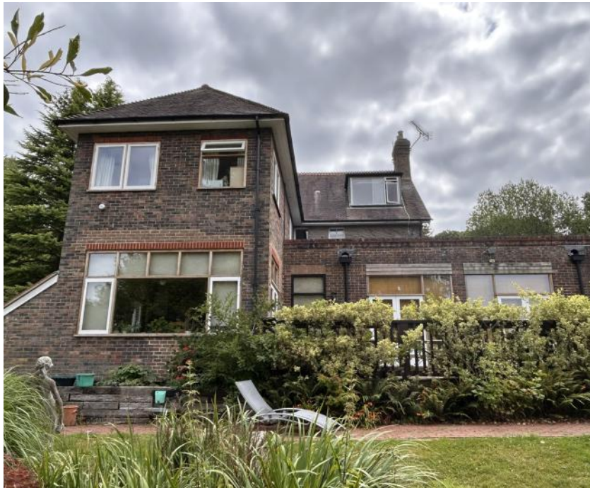
Rear of house from the garden, with flat roof visible on the right of the image. The box dormer is visible above.
