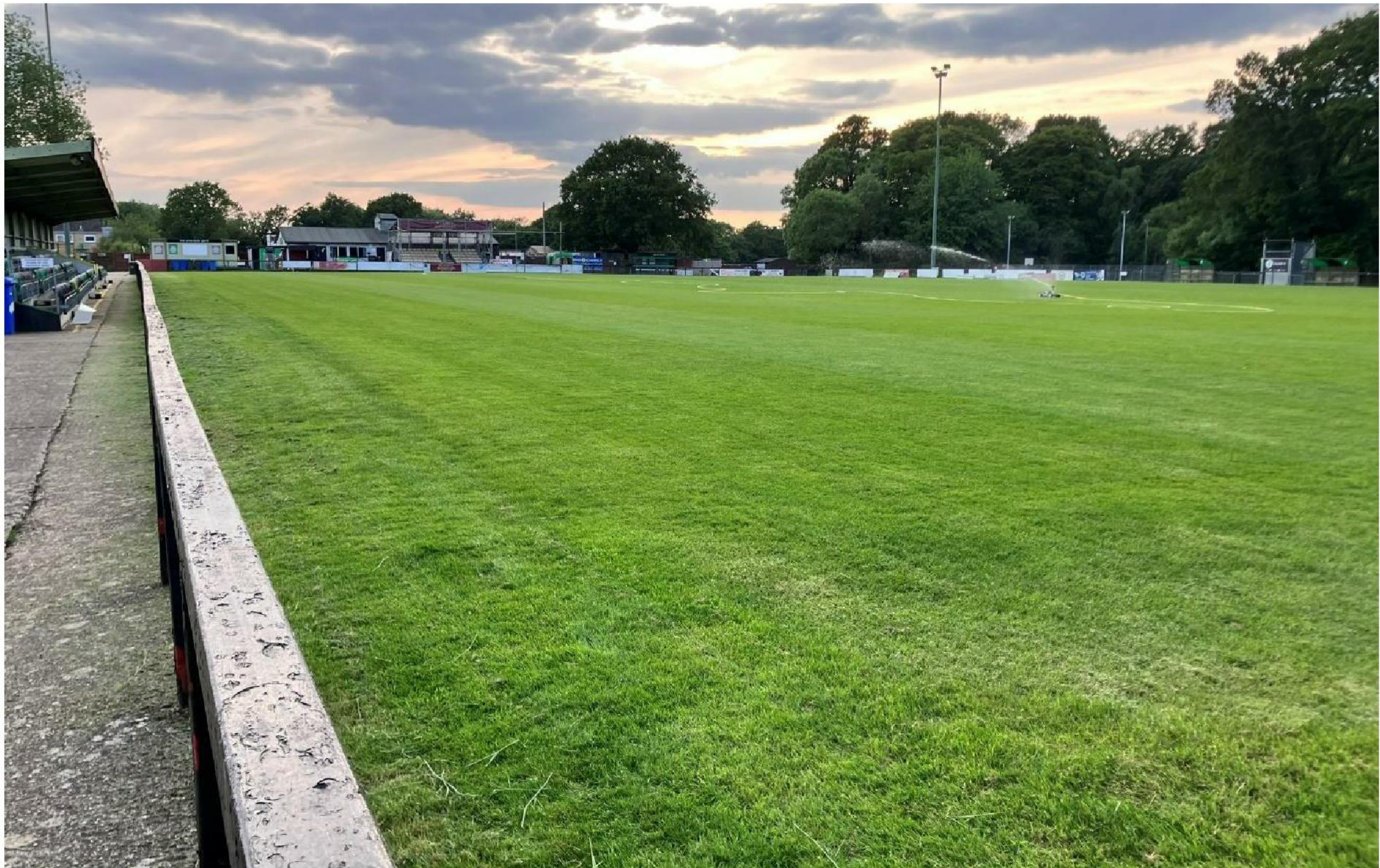
Photograph 1: showing the existing football pitch, with the metal fence boundary and concrete surrounds with areas for small stands.
