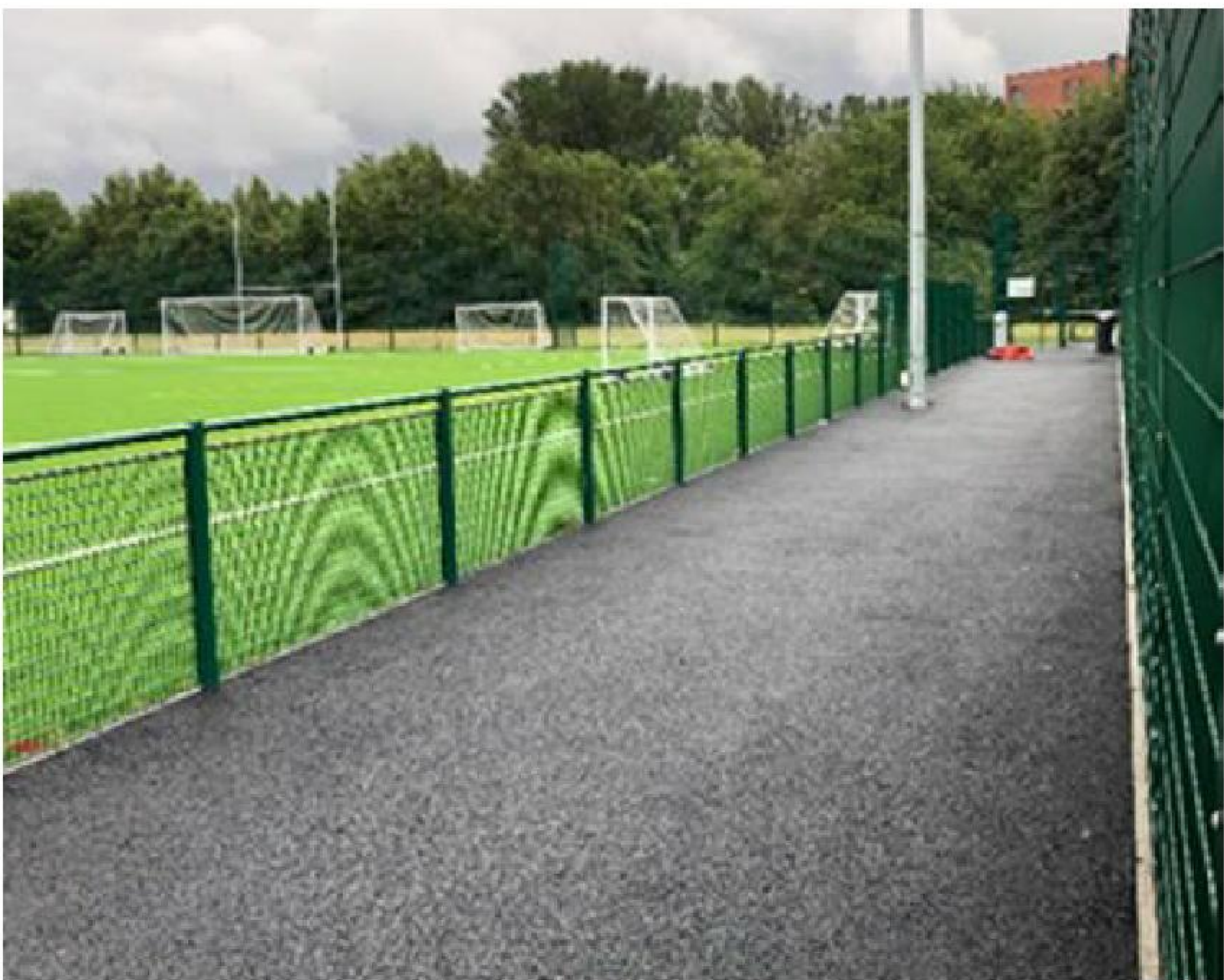
Typical example of ball stop fencing
