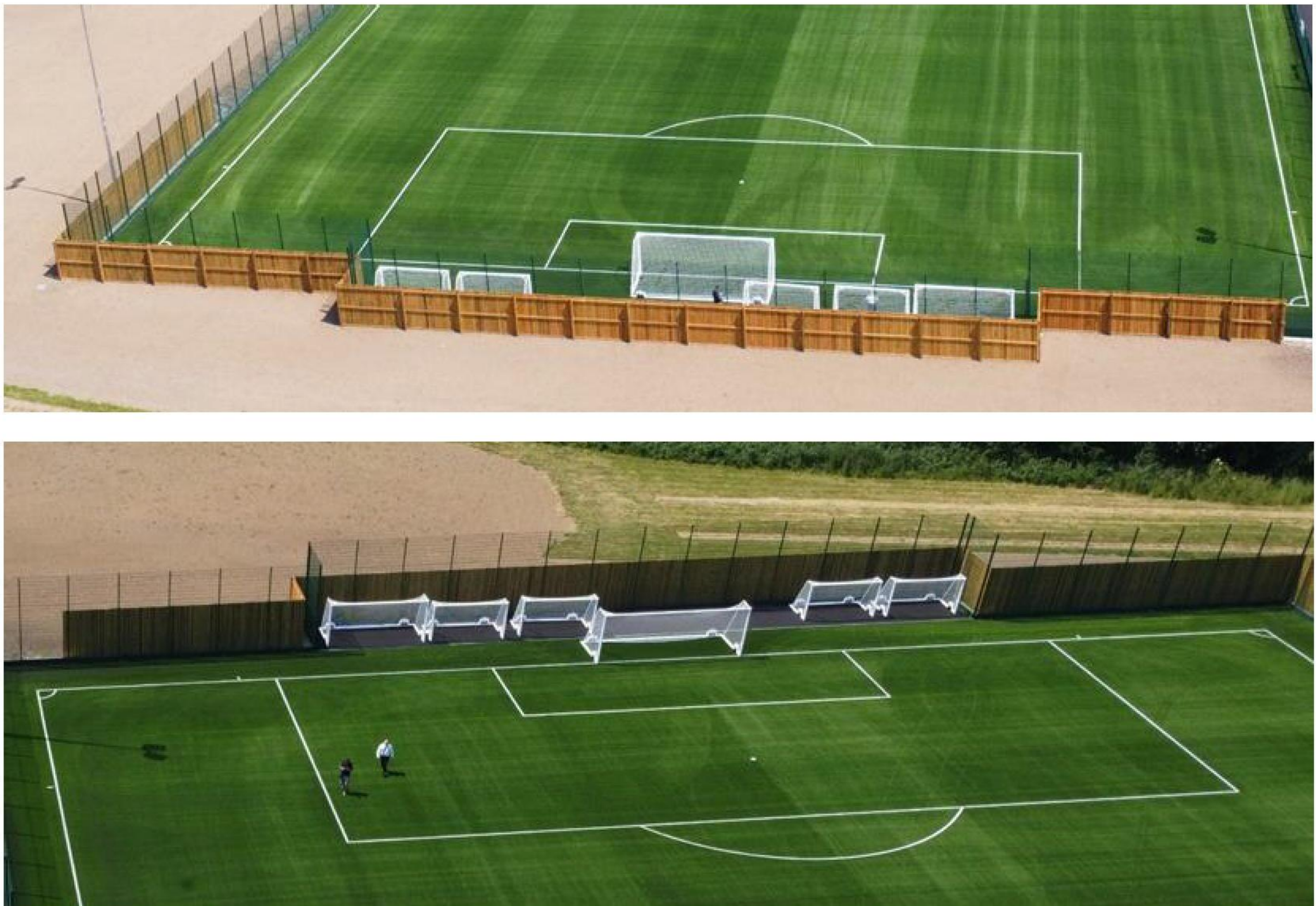
Example of perimeter acoustic fencing
