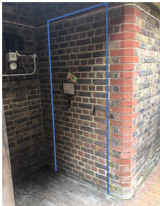
Figure 4: Re-instated Doorway to fuel store
