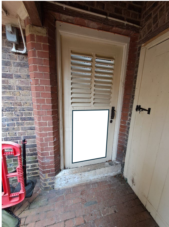
Figure 5: New location of matching door louvre window
