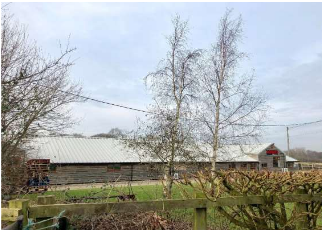
Fig 3: The existing commercial building located immediately to the north of the proposed site dates from the 1970's and consists of a metal roof with timber cladding.
