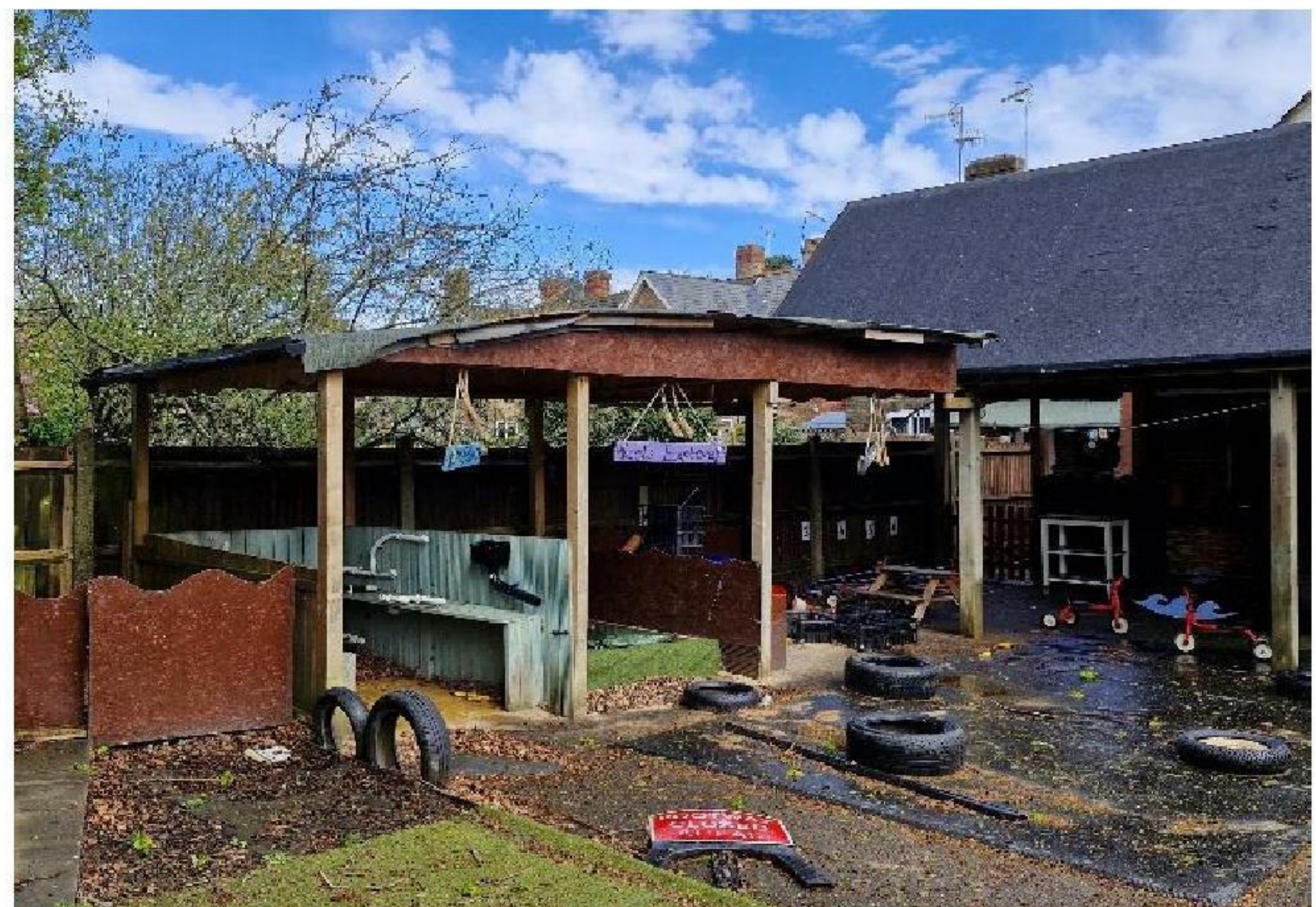
Figure 3 - Proposed location of new shelter (structure demolished)
