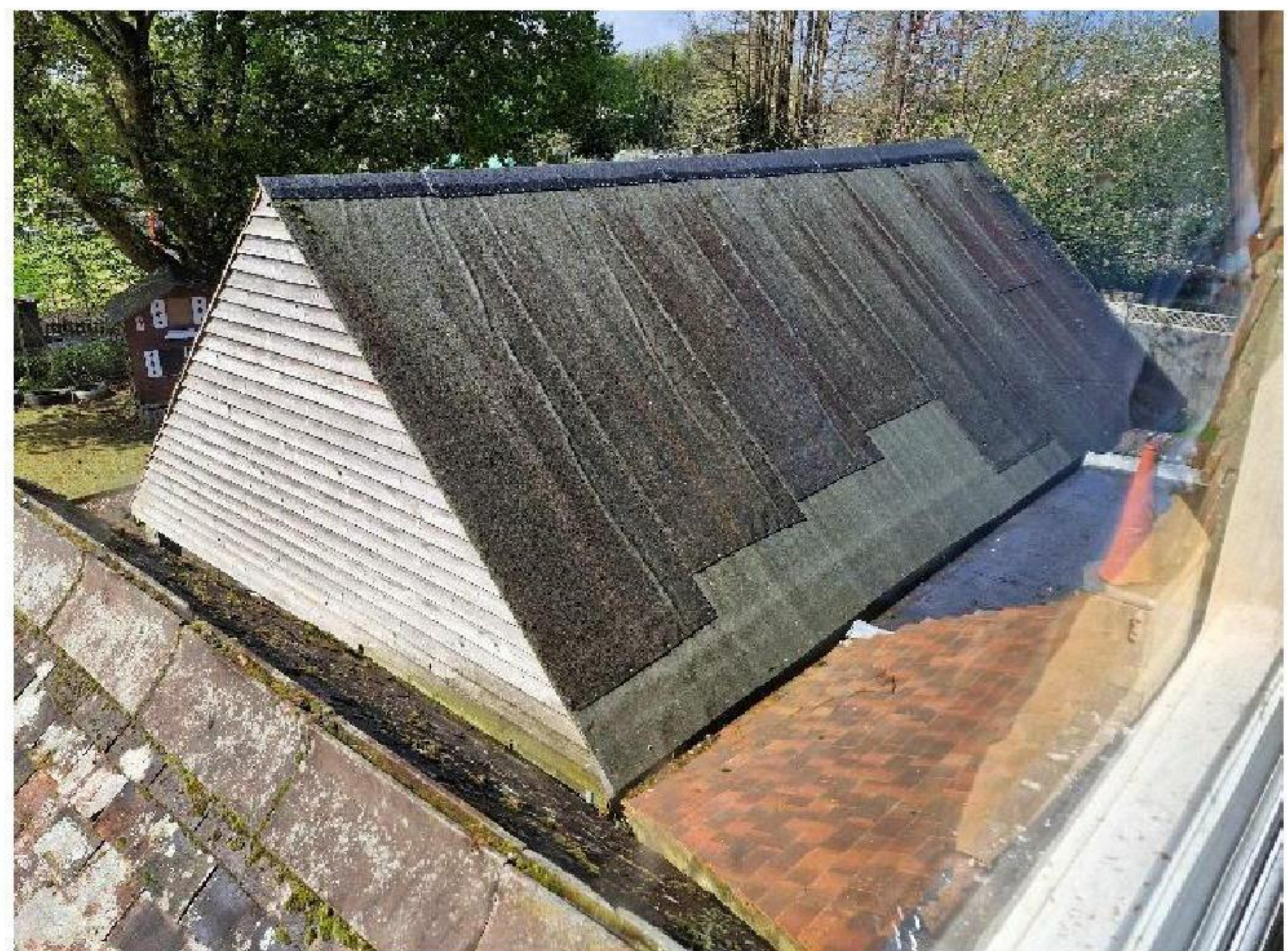
Figure 3 - Previous structure roof (now demolished)
