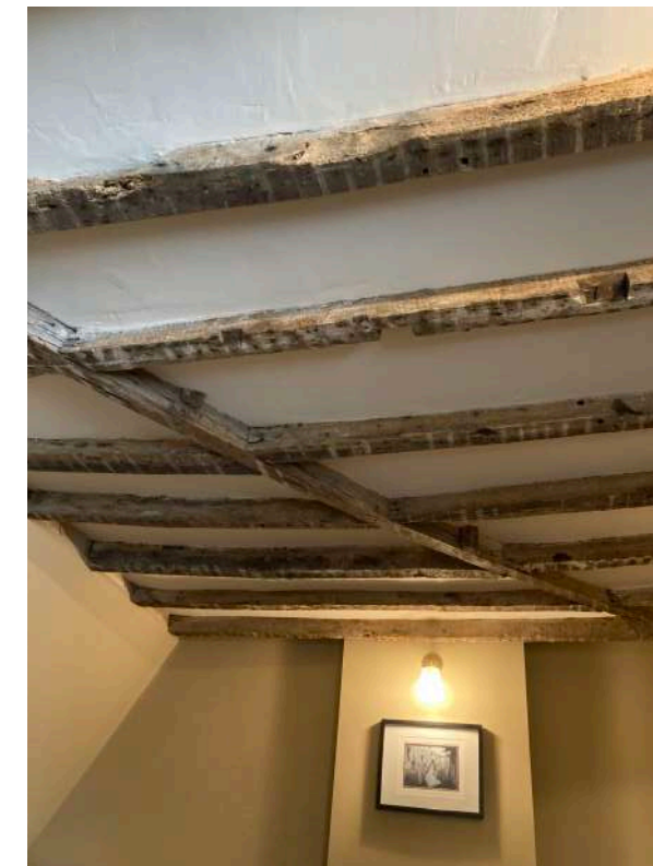
Exposed beams to attic (left) and main bedroom (right)
