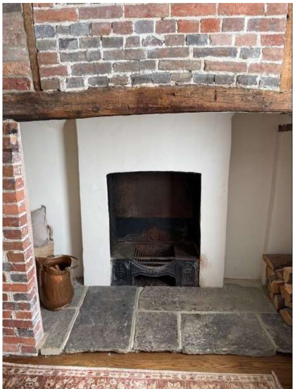
Former inglenook fireplace to ground floor living room at east end of 4 Ivy Cottages
