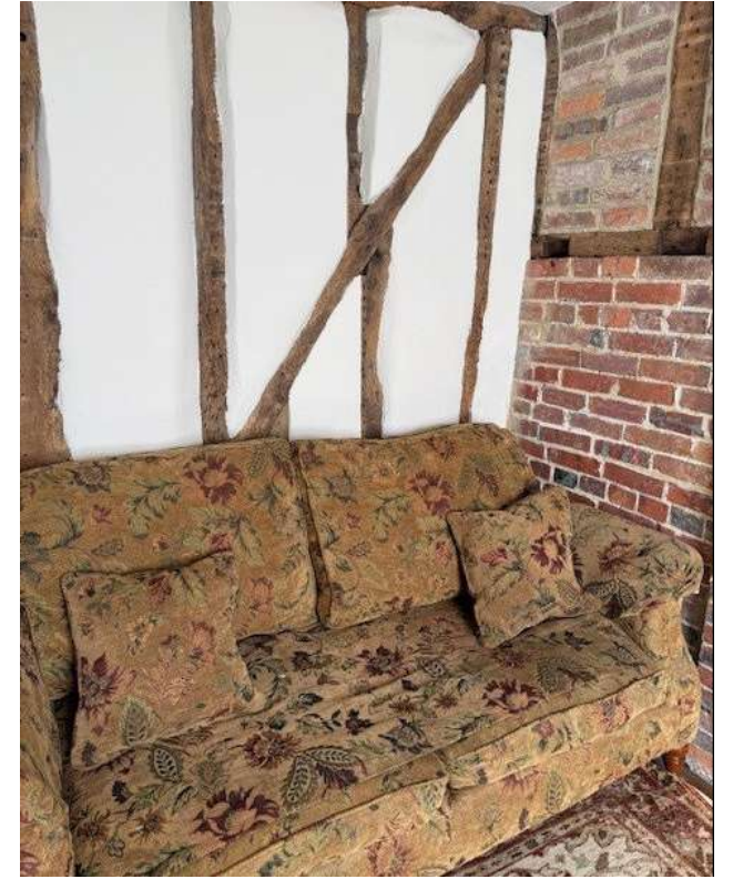
Timber framing to living room looking towards kitchen
