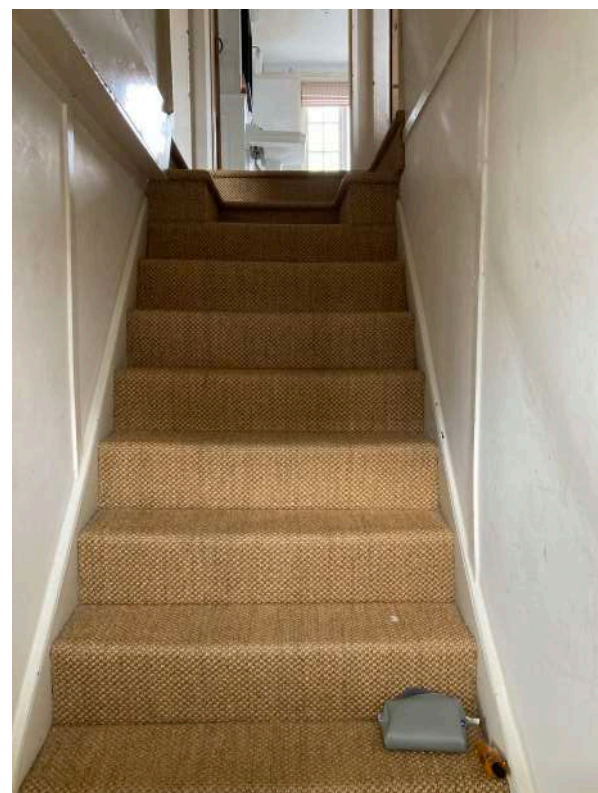
Staircase from ground to first floor
