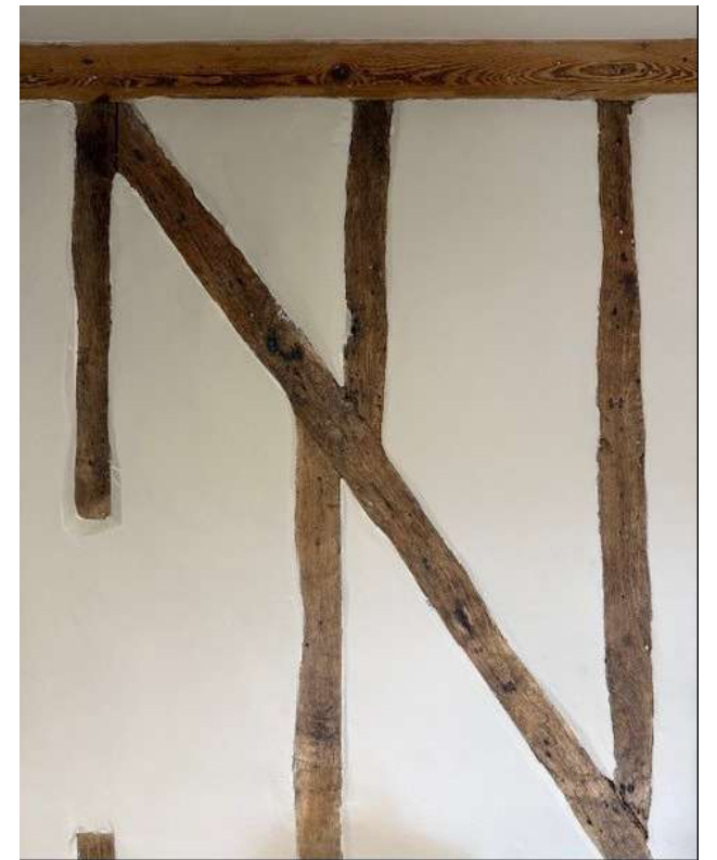
Timber framework to kitchen
