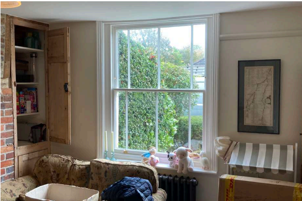
Example of sash window of re-fronted south elevation of 4 Ivy Cottages
