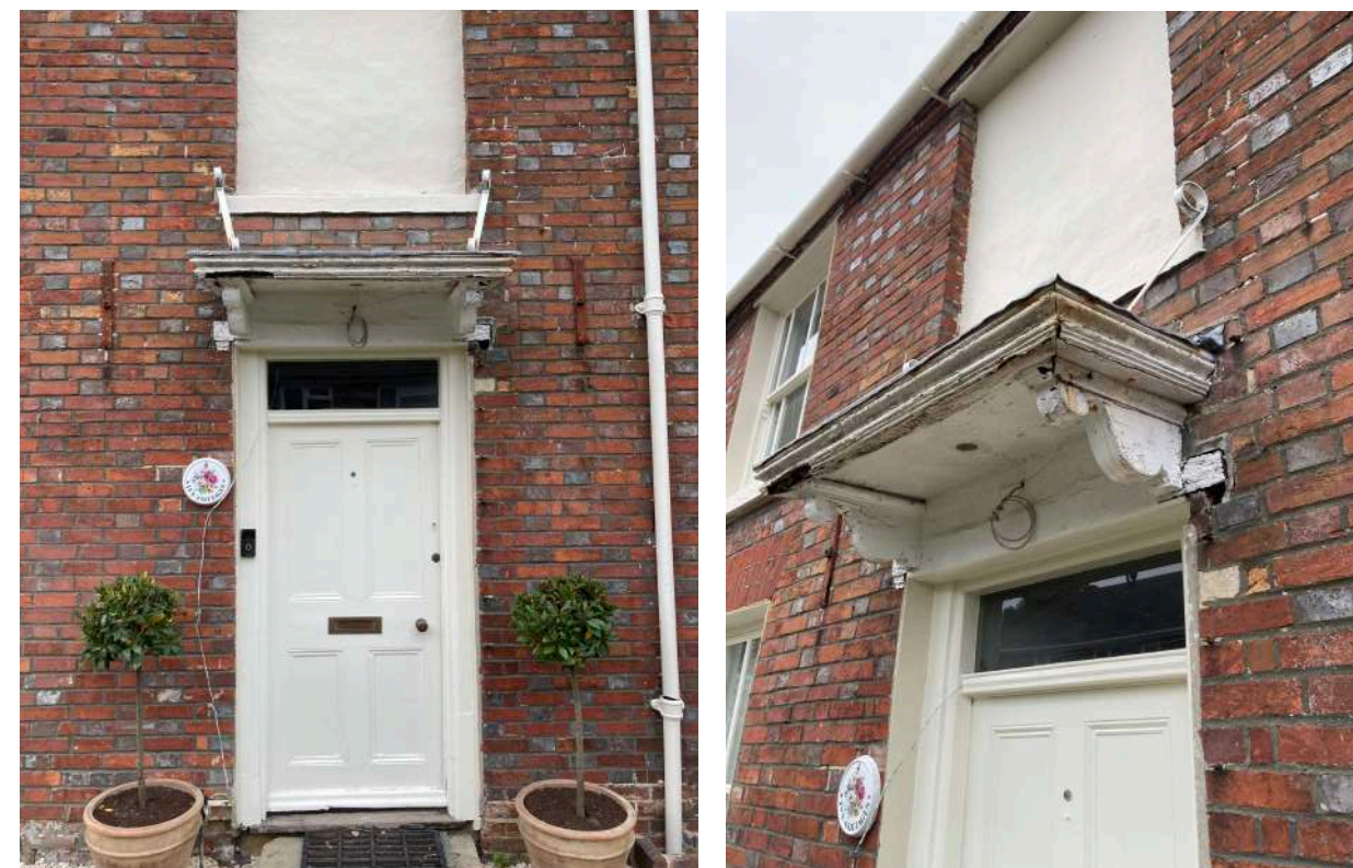
Existing canopy above front door, south elevation, with detail of brackets
