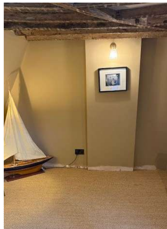
Exposed ceiling beams to attic space
