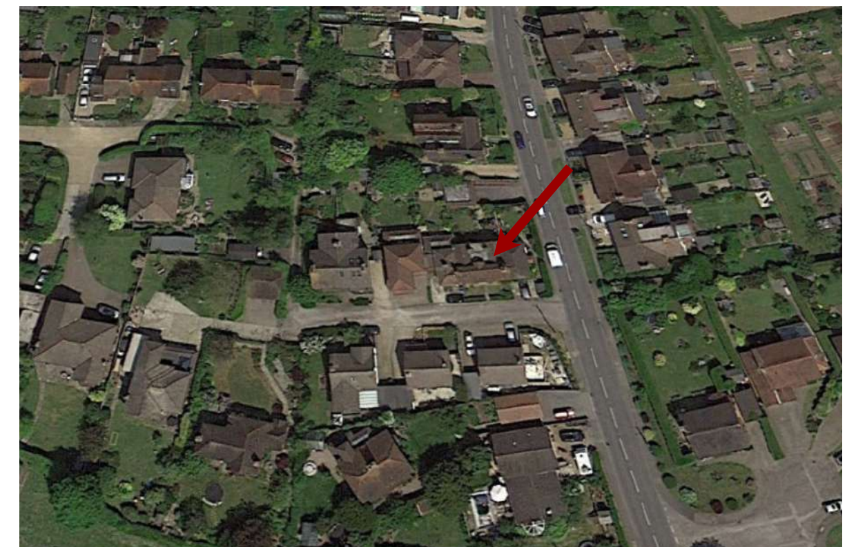
Aerial imagery, 2013 illustrating location of Ivy Cottages (Google Earth Pro)
