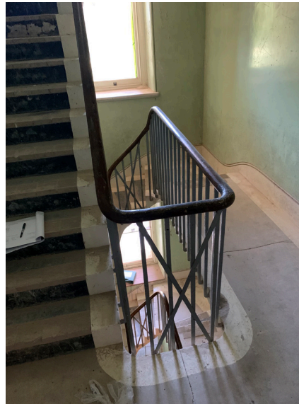
Example of existing stairwell balustrade retained
