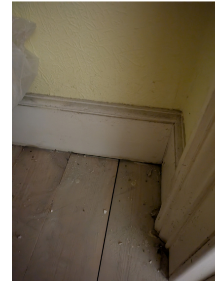
Original skirting to S18
