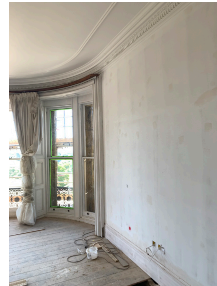
Example of cornicing and skirting retained
