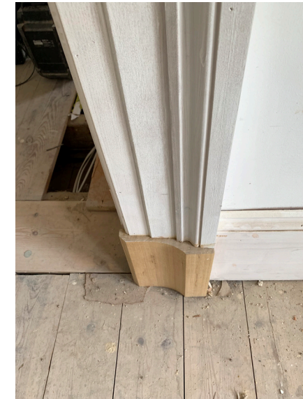
Example of door and skirting detail
