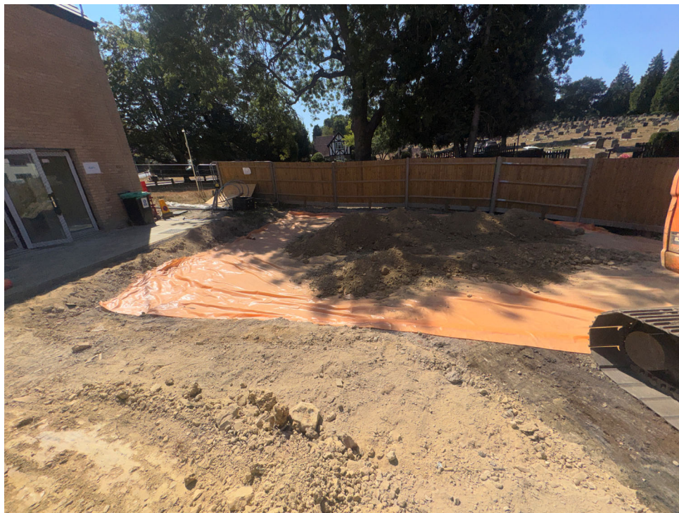
Photograph 4: Placed materials within Plots 1 and 2 over geotextile.
