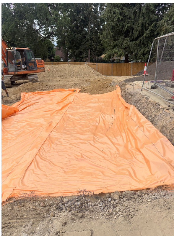
Photograph 2: Placement of clean materials over geotextile within Plots 5 and 6.
