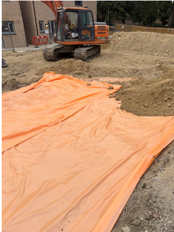
Photograph 3: Placement of clean materials over geotextile within Plots 3 and 4.
