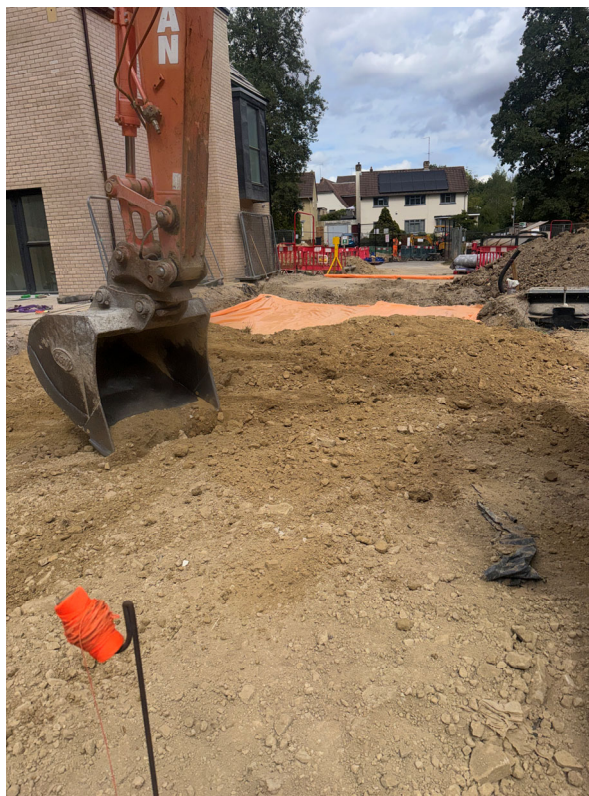
Photograph 1: Placement of geotextile and clean materials between Plots 7, 6 and 5.
