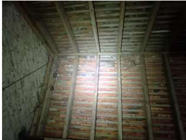
Fig. 9. – View to roof ridge of stable
