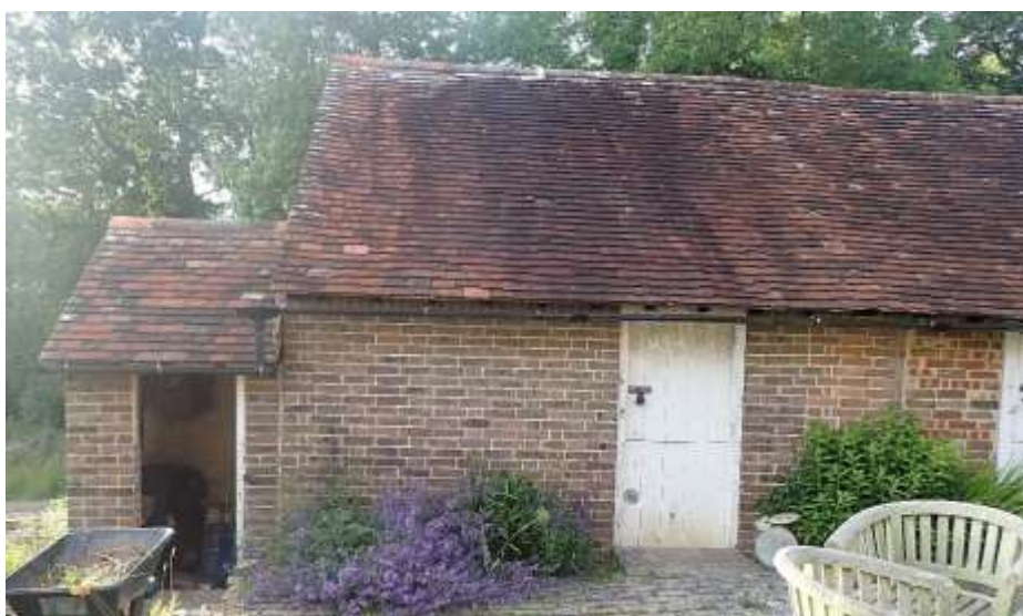
Fig. 1, View of SW of former stable
