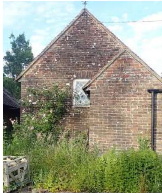
Fig 3 – Outbuilding, viewed from W end
