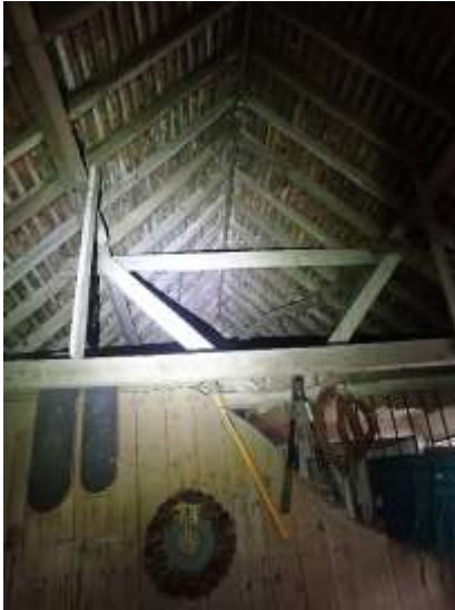
Fig. 5 – Interior of stable, looking towards E
