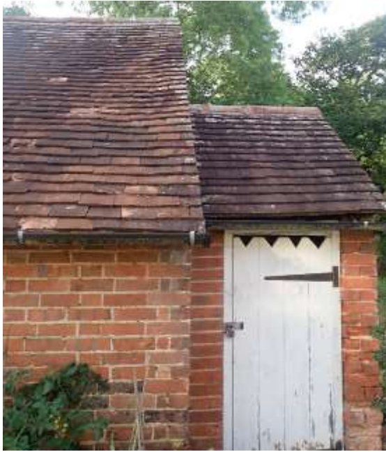
Fig. 2 - SE end of former stable
