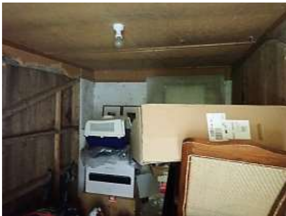
Fig. 7 – View of E section of stable, with ceiling board above
