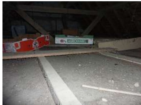
Fig. 8 – View across ceiling board
