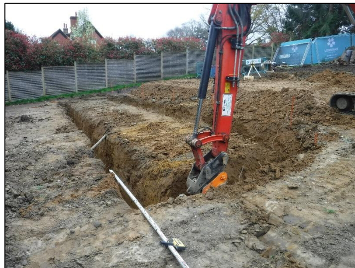
Plate 1: Excavation of footings.
