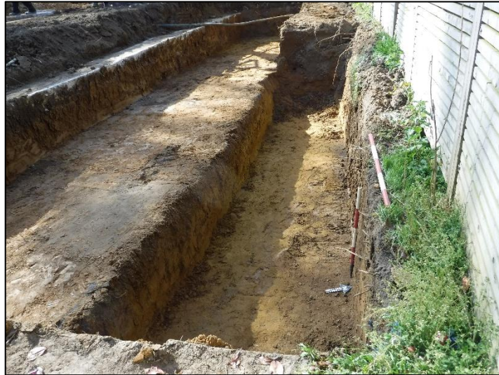
Plate 5: Showing terraced soakaway excavations.
