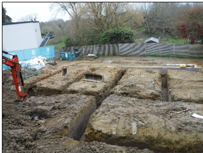
Plate 3: Looking North showing the completed footings.
