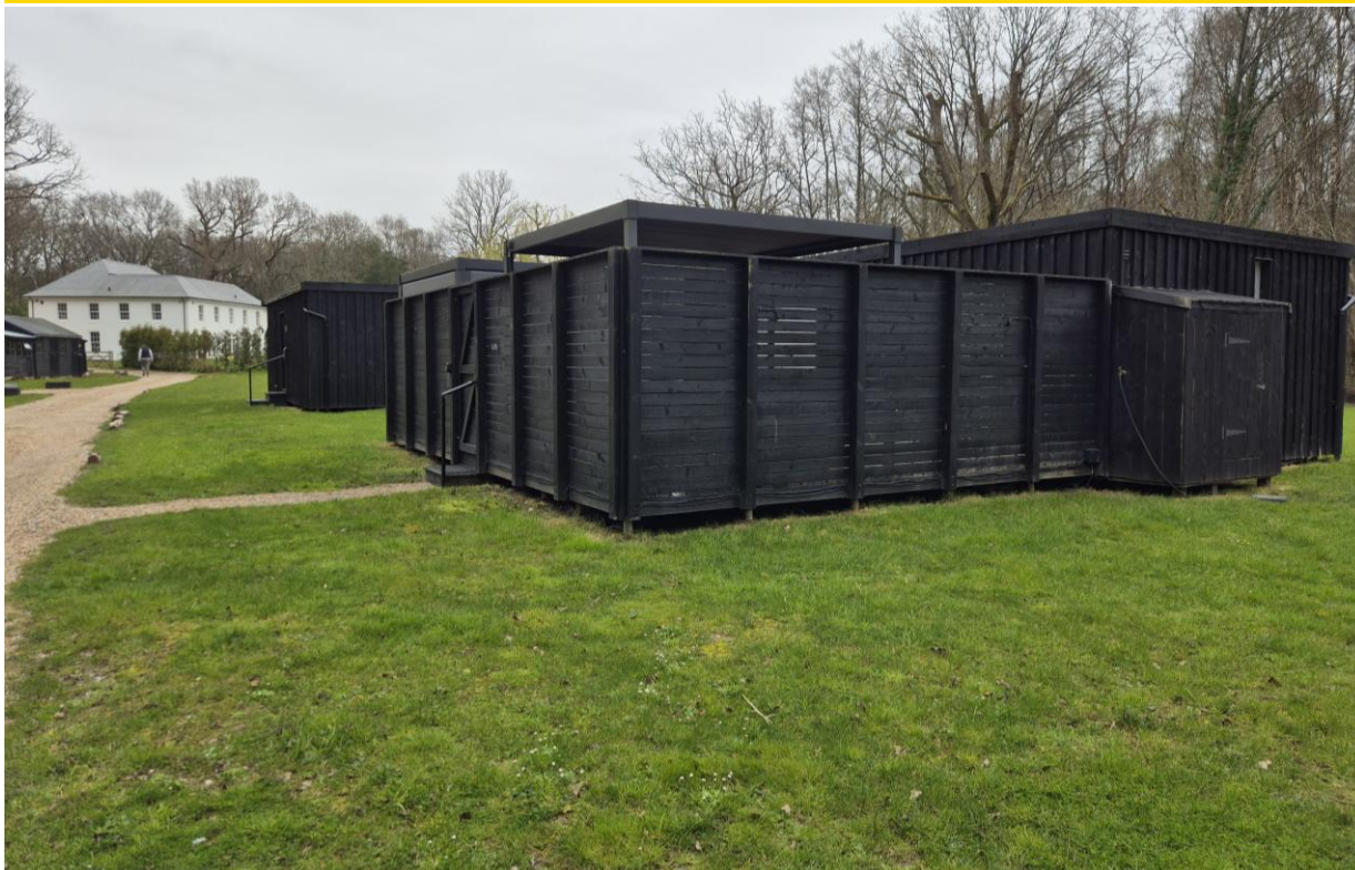
The existing cabins, viewing east.
