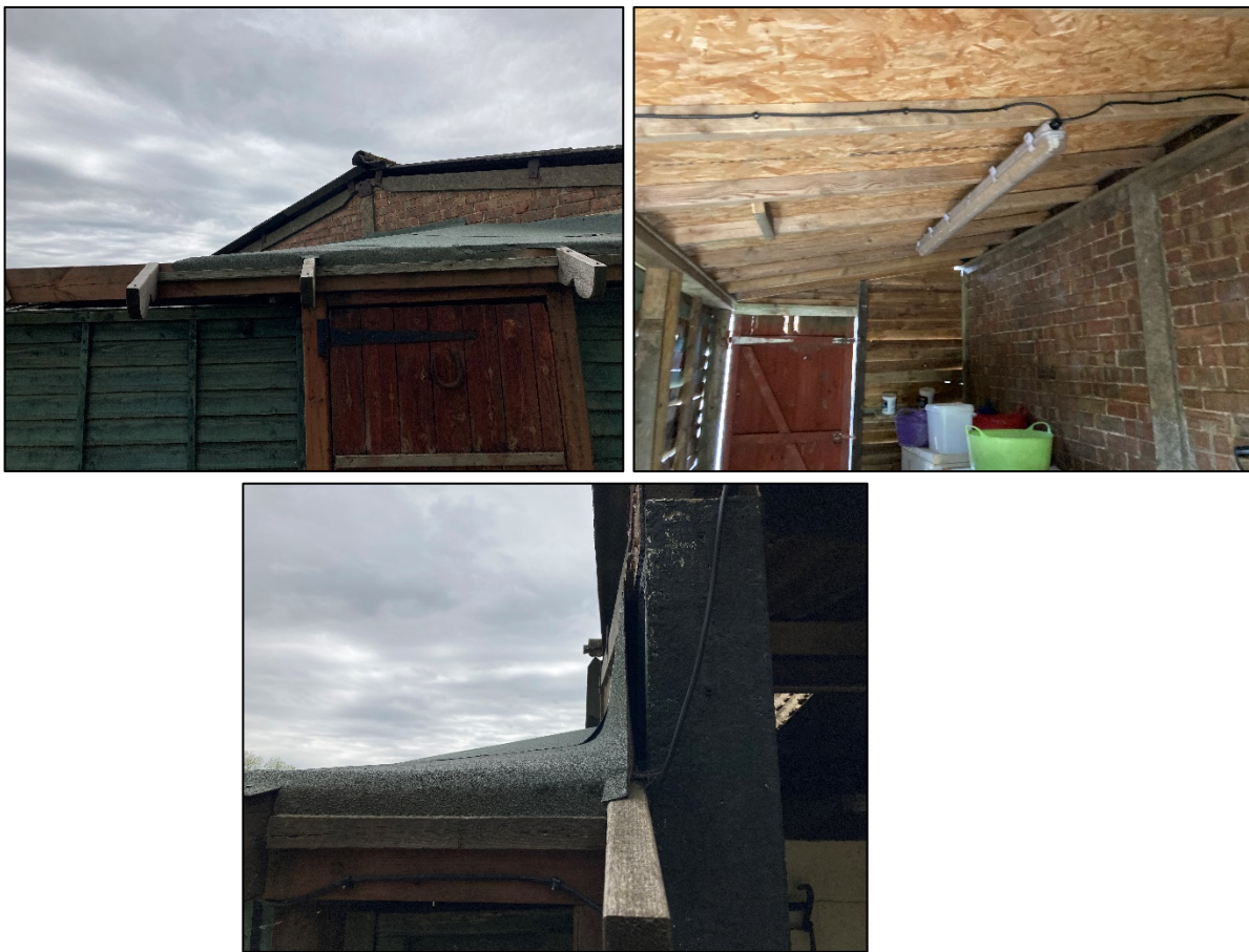
Photograph 4. The attachment of a further storage area on the south elevation. Note the gap where it joins the existing stables.
