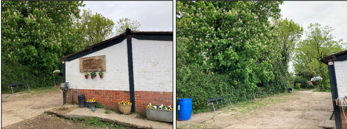
Photograph 1. The north elevation looking towards the east boundary. Note the location of a small woodland parcel adjacent to the site.
