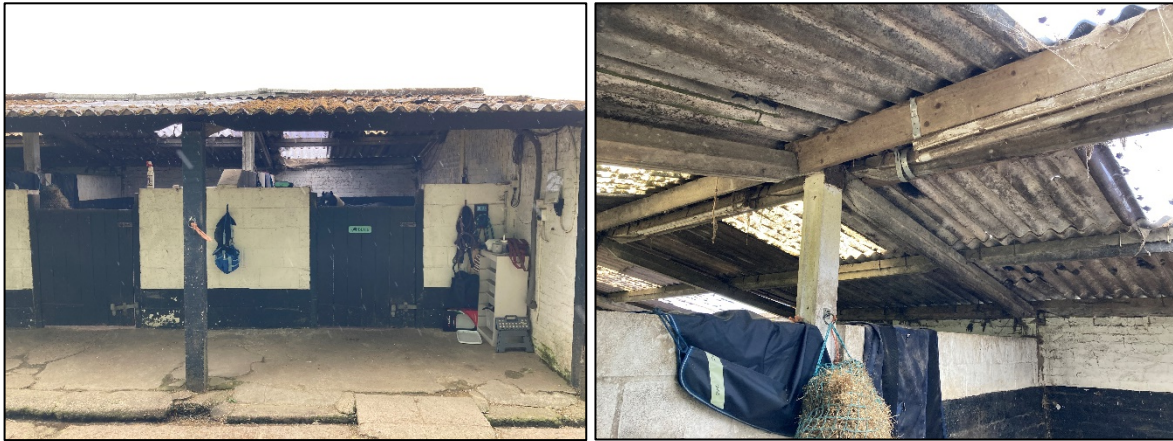
Photograph 3. The eastern elevation of the stable block. Note the internal cobwebbing and lack of cracks or crevices.
