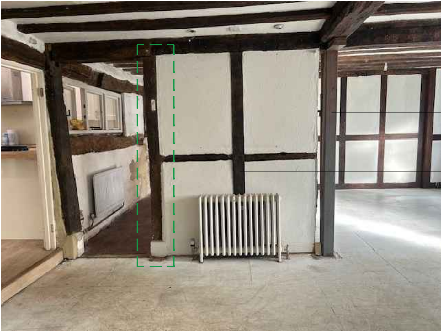
Internal lounge wall prior to changes.
