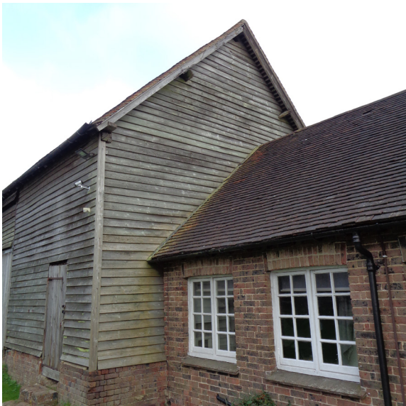
Rear (West Facing) Elevation
