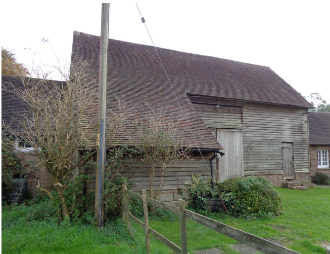
Rear (West Facing) Elevation
