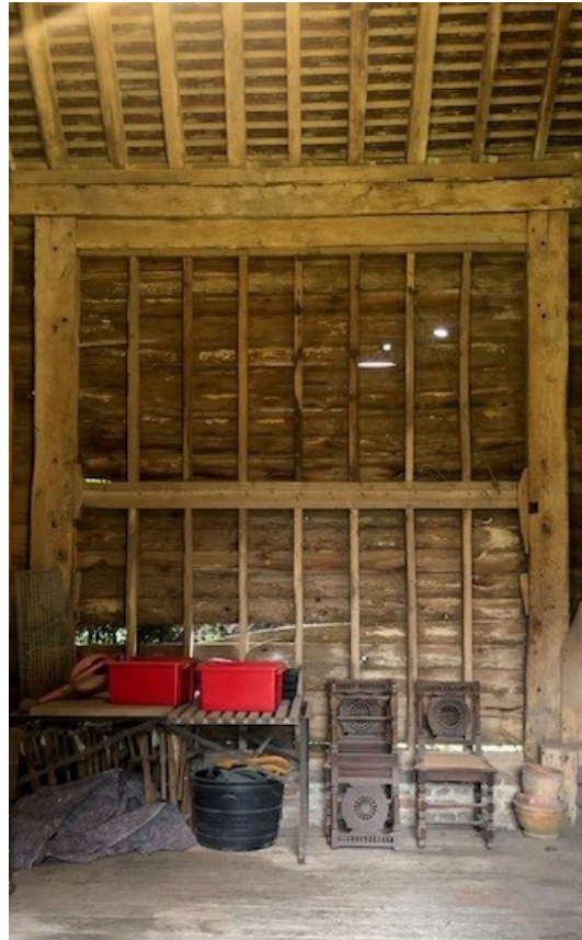
Retain internal exposed timber aesthetic and timber threshing floors.
