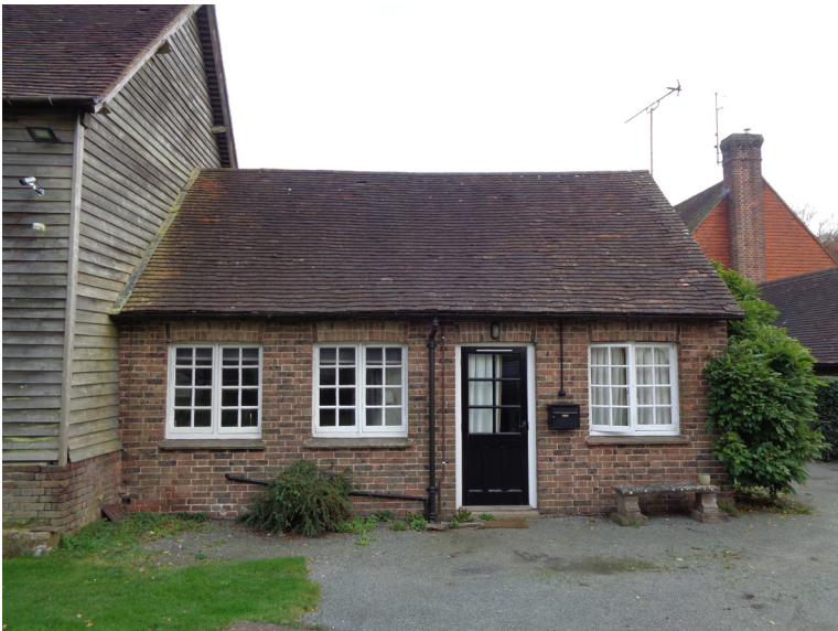
Rear (West Facing) Elevation
