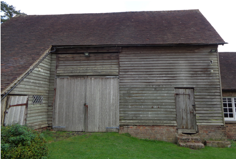
Rear (West Facing) Elevation
