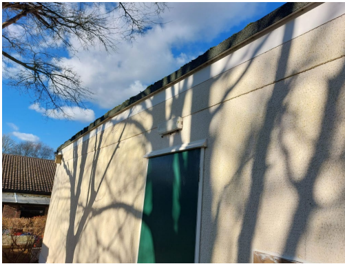
Image 16: View of B03, showing the felt roof lip surrounding the roof, providing roosting opportunities.
