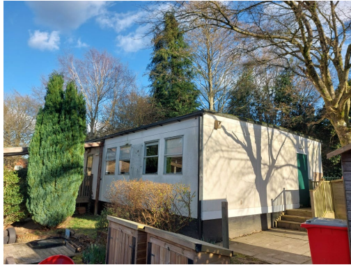
Image 01: Northwest corner of B03.
