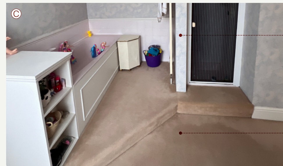
ROOM F12 - BATHROOM
