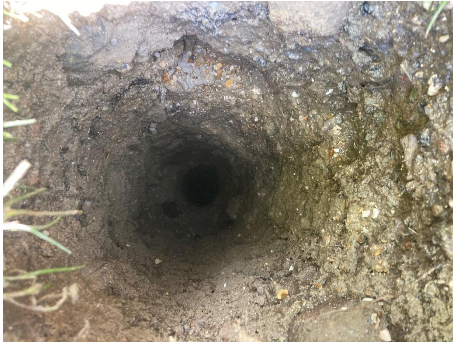
P10: Photograph showing inspection pit from BH02.
