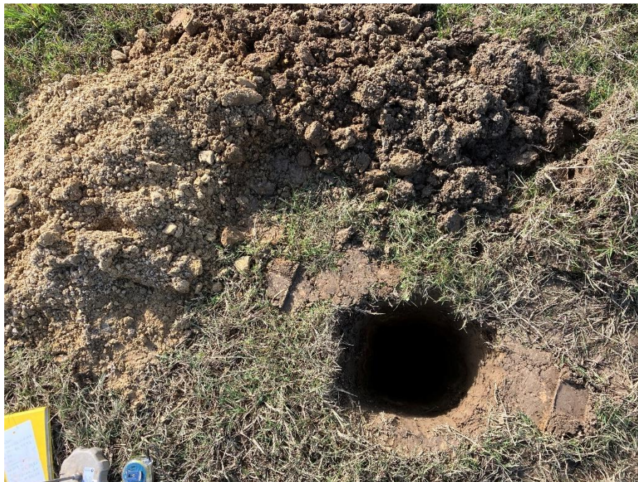
P8: Photograph showing contents of inspection pit of WLS03.
