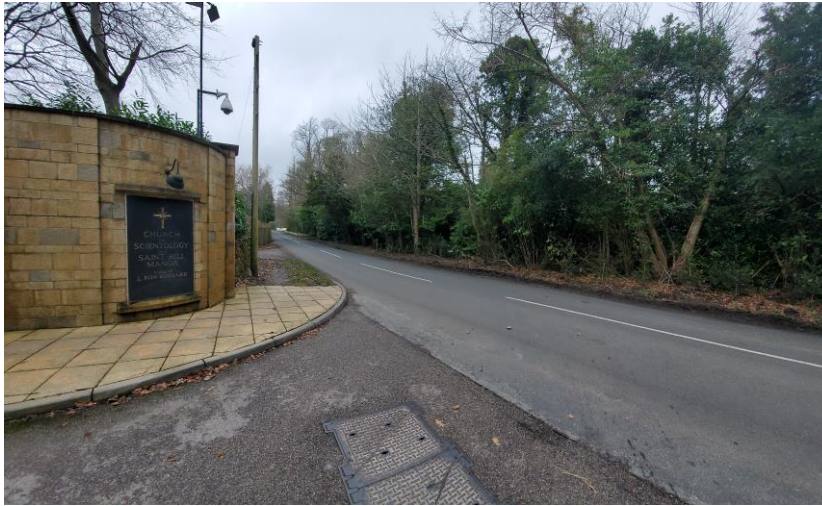
Figure 2.9 Southern access (North Gate) looking north
