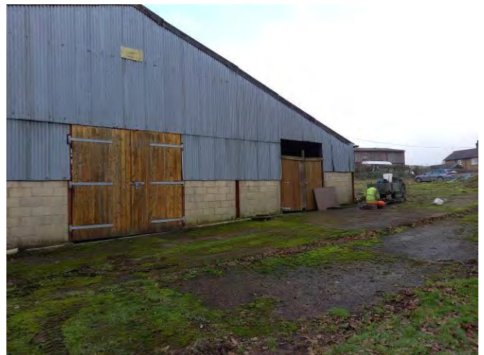
Existing structure on site.
