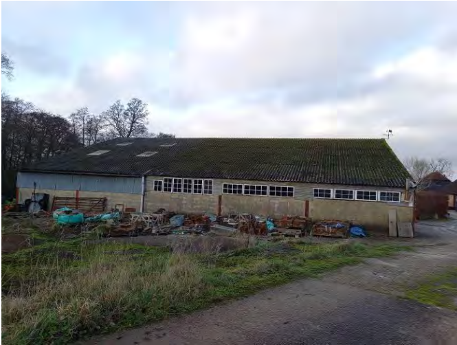
Existing structure on site.
