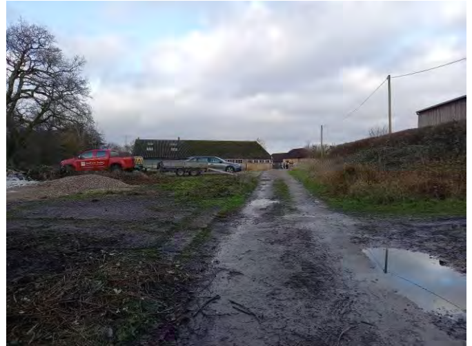
View from south east of site looking north.
