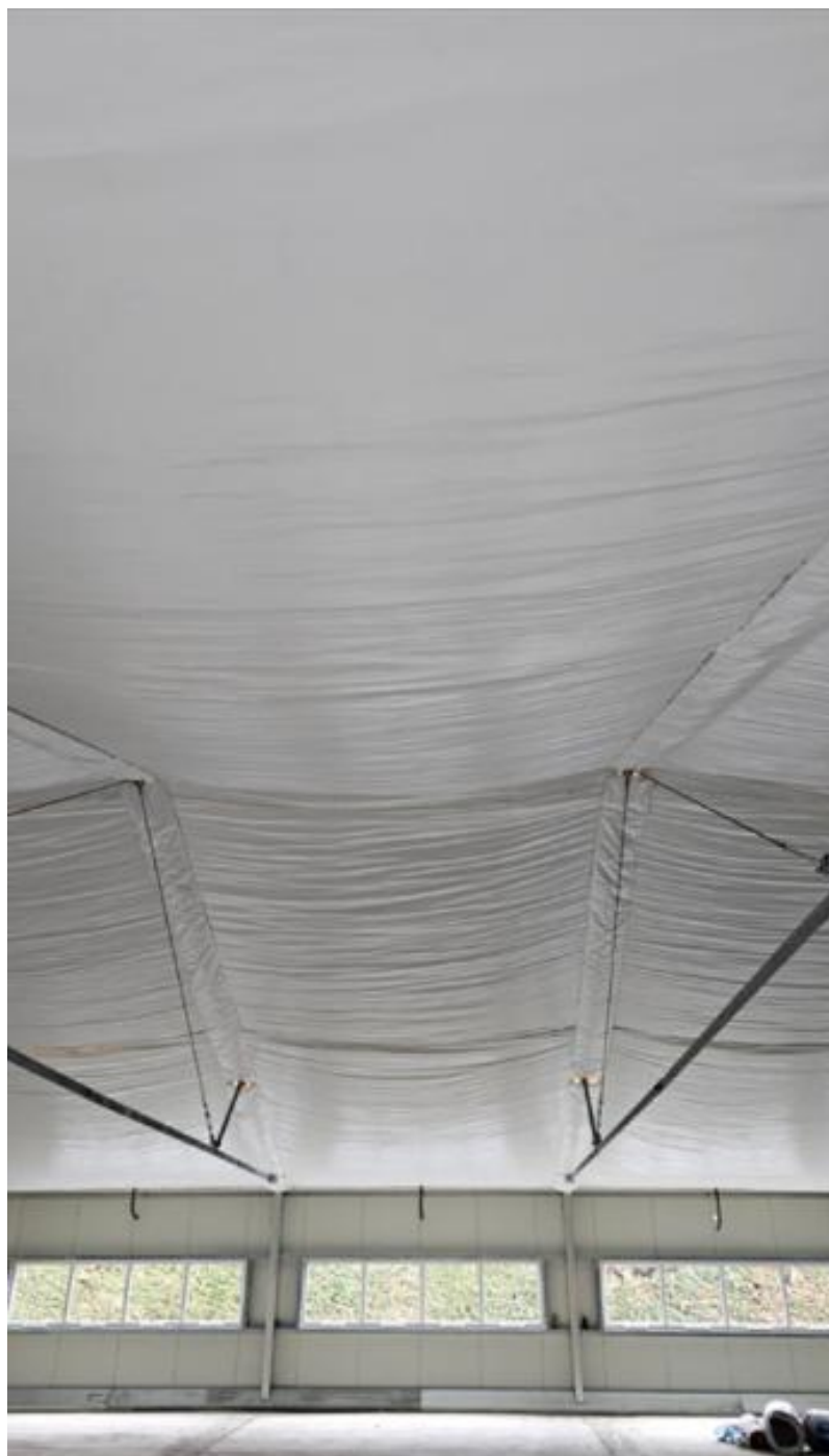
Figure 6.2: Example of MAL22 acoustic lining applied to the underside of a canopy structure
