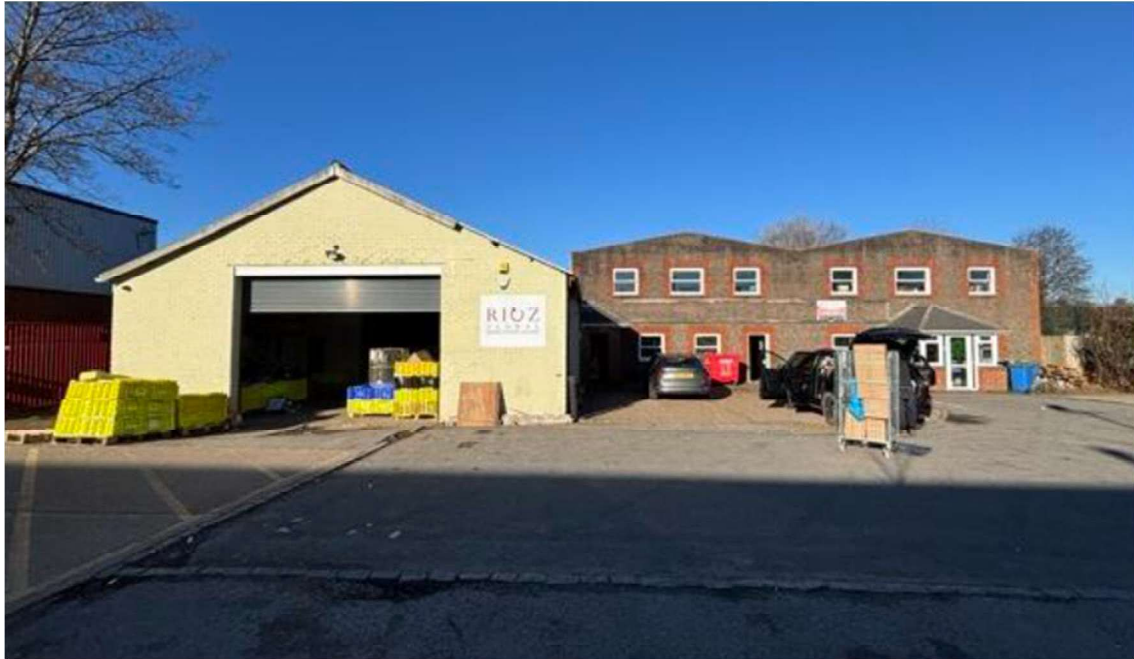
Figure 8: Units 3 and 4 School Close Site
