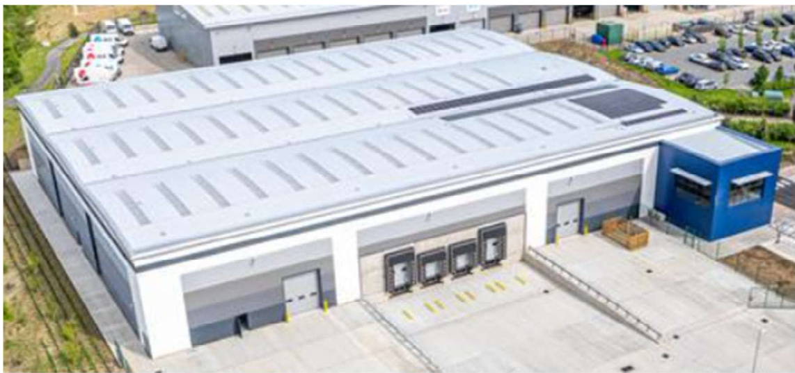
Figure 15: View of Unit 3 at Panattoni Park
