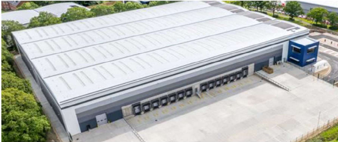
Figure 16: View of Unit 7 at Panattoni Park
