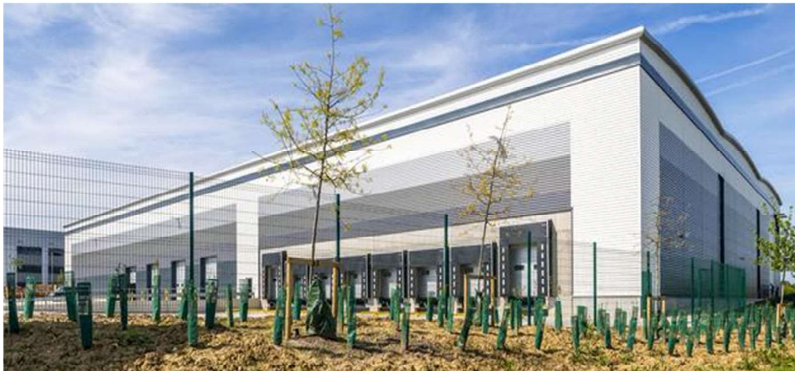
Figure 14: View of Unit 1 at Panattoni Park
