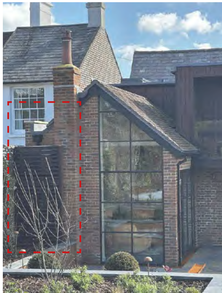
Recent photograph capturing the new AC AHU louvred enclosure on the rear of the bake house
