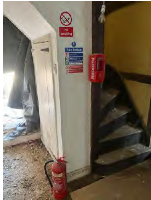
Staircase during demolition works
