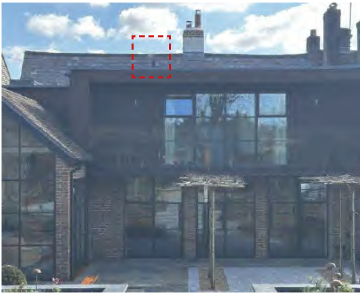
Recent photograph capturing the new boiler flue
