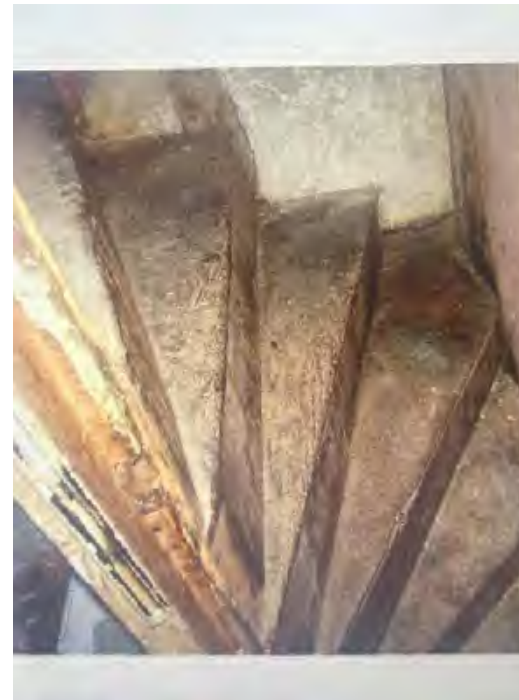
Staircase during demolition works
