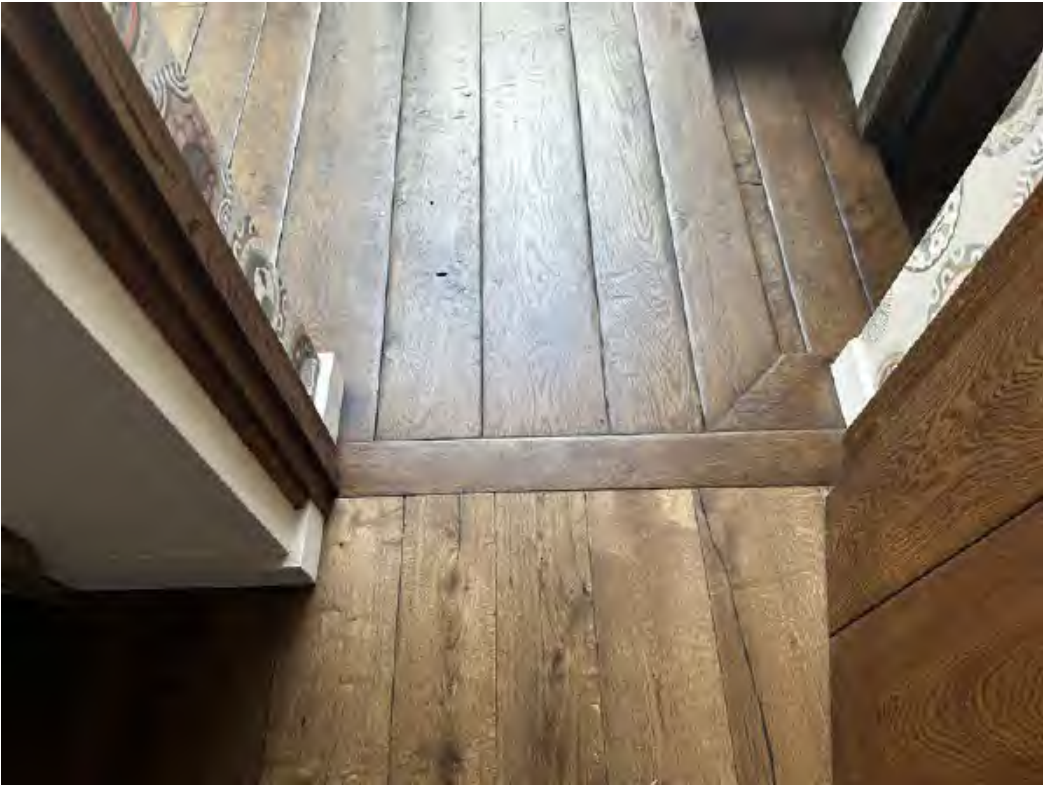
As-built oak flooring
