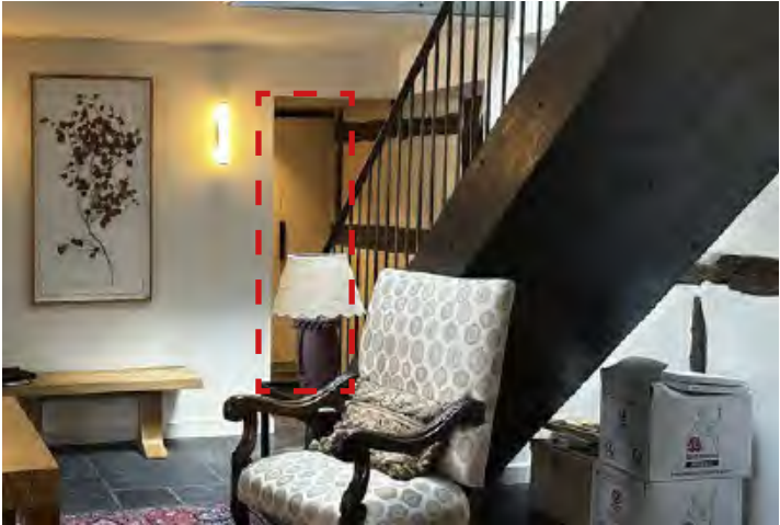
Photograph showing location of the door
