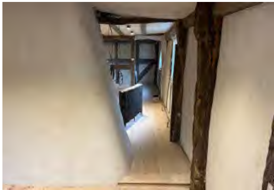
Pre-construction photograph of space between bedrooms, walls re-rendered prior to installation of fitted wardrobes
