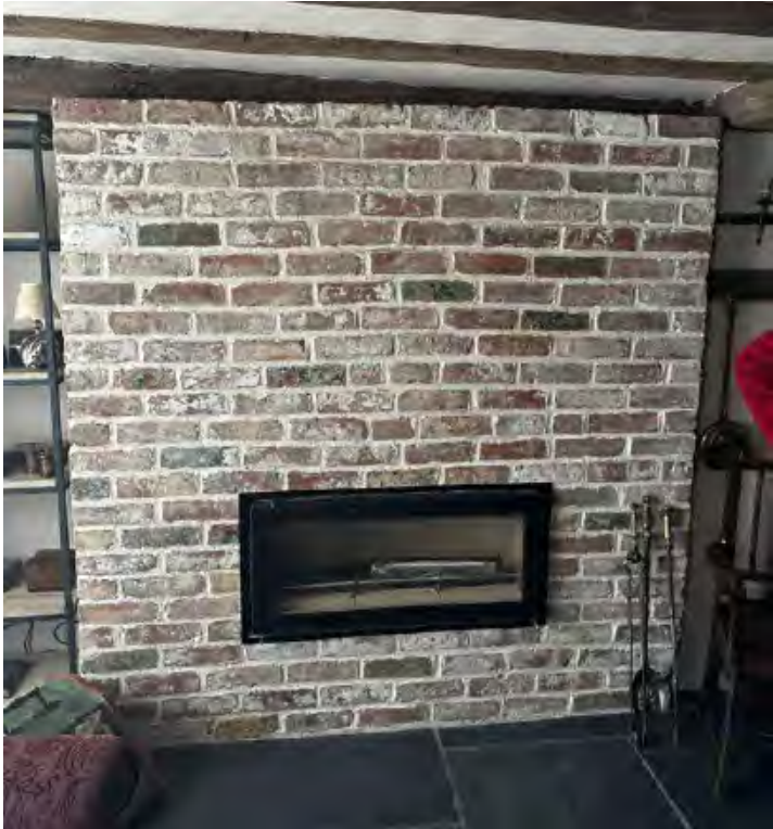
Ground floor living room re-faced chimney breast
