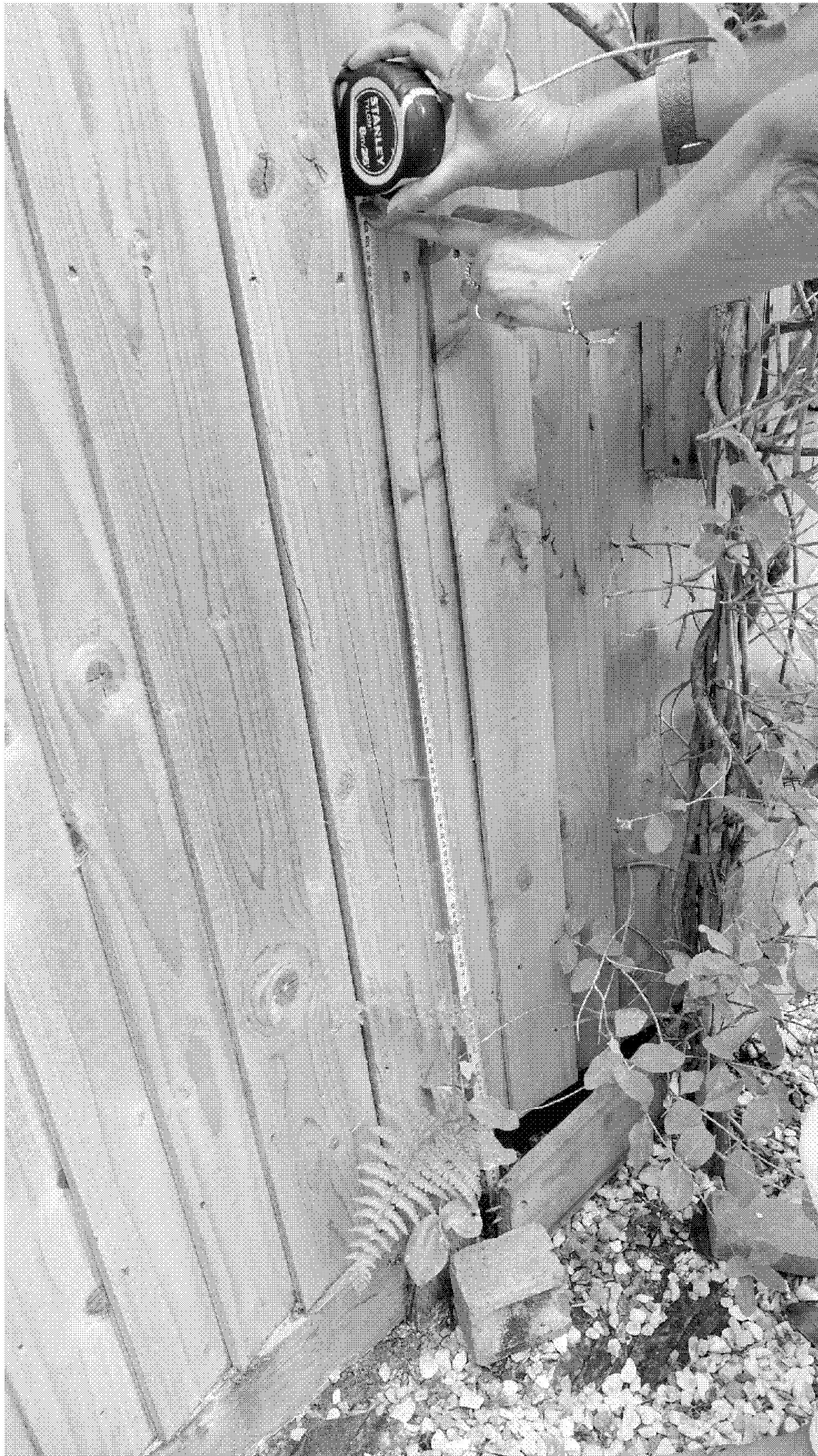
Figure 6: Tape indicates increased height of the ground level post land raising
